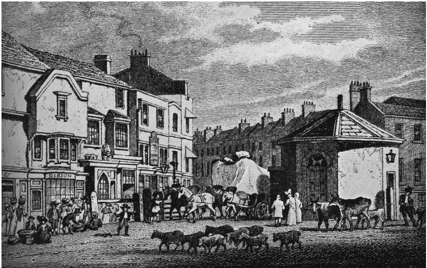
Islington Toll Gate (1829)
