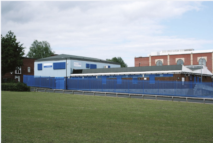
Figure 6.3 Doctor's surgery on the boundary of Neighbourhood B. Defensive measures include a 2m spiked fence, spiked anti-climb rollers, and armoured doors and windows. Image © Daniel Nettle, CC BY.
