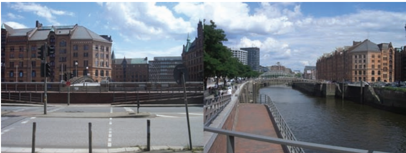
Figure 3: Existing flood defences along the Customs Canal and their utilisation as viewing points
