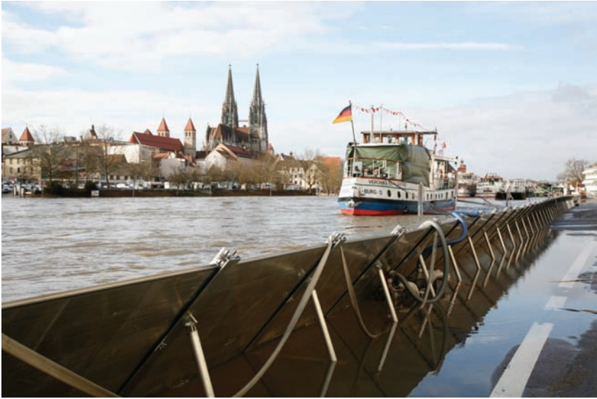
Figure 2: Mobile Flood-Walls in the Old Town of Regensburg and Stadthof
