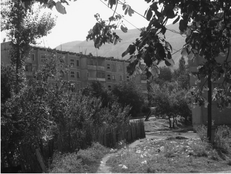
The five-story apartment buildings in the center of Kokjangak, August 2009
