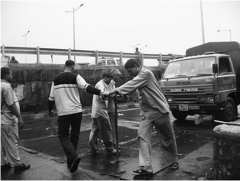
FIGURE 6. Two pairs of chaviwallas turn the valves of underground city water pipes while the mukadam (foreman) looks on.
