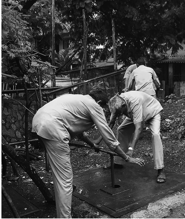
FIGURE 1. Chaviwallas turning a valve on city streets. All photos are by the author unless otherwise credited.
