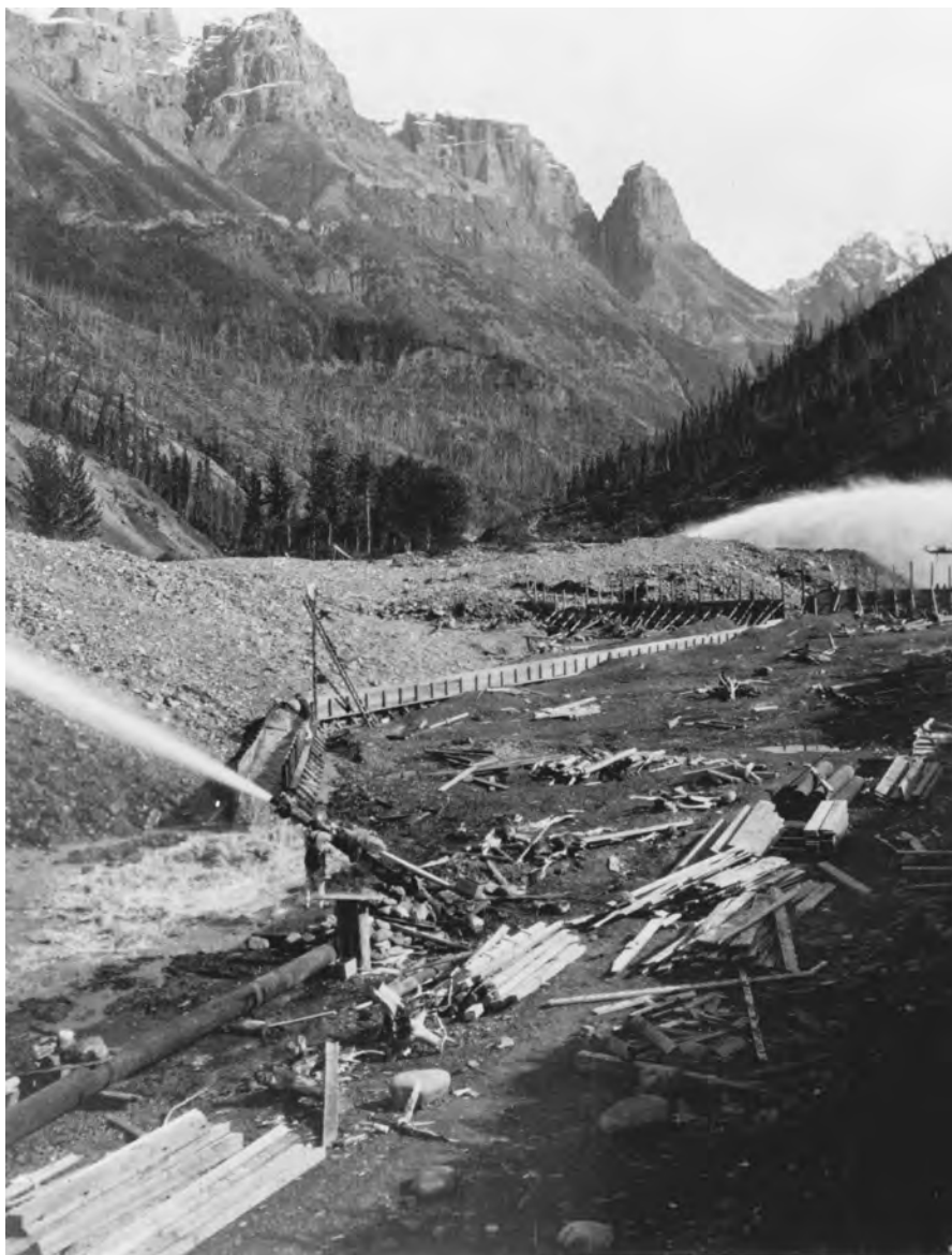
Hydraulic mining operation on Dan Creek, a tributary of Nizina and Chitina rivers in the Wrangells. Alaska files 8268, University of Washington Archives. Hydraulic mining escalated the impact on the land.
