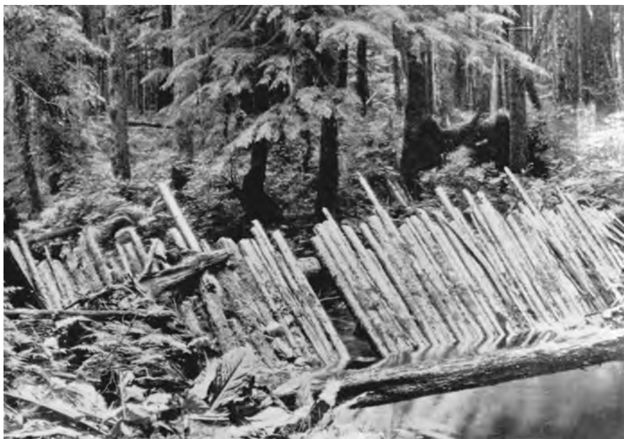
Dam on salmon stream, Helm Bay, ca. 1898. In Jefferson B. Moser, The Salmon and Salmon Fisheries of Alaska, Washington, DC: GPO, 1899, plate 10. Early commercial fishers blocked streams to maximize their catch, damaging salmon populations in the process.
