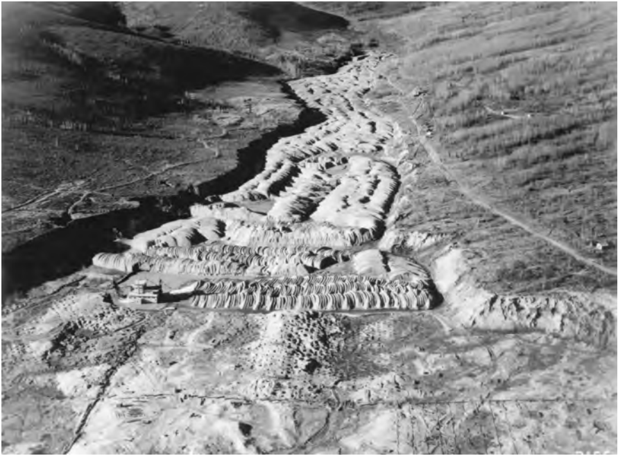
Fairbanks Exploration Co. dredge on Cripple Creek, twelve miles from Fairbanks. Alaska files 8272, University of Washington Archives. Such large-scale operations could permanently alter an entire valley.
