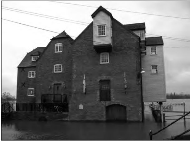
Figure 2. Tewkesbury Abbey Mill in Flood, May 2021. Mill Bank itself has a raised walkway along the east side of the Mill Avon, on which a range of timber framed houses sit. The walkway has historic origins but was refaced in the 19th century in blue engineering bricks, retaining the original stone steps on Mill Street.
