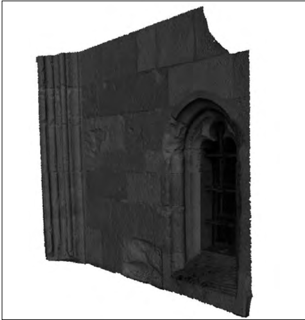
Figure 14. Photogrammetry of the exterior of Winchester Cathedral, the ERT study area.
