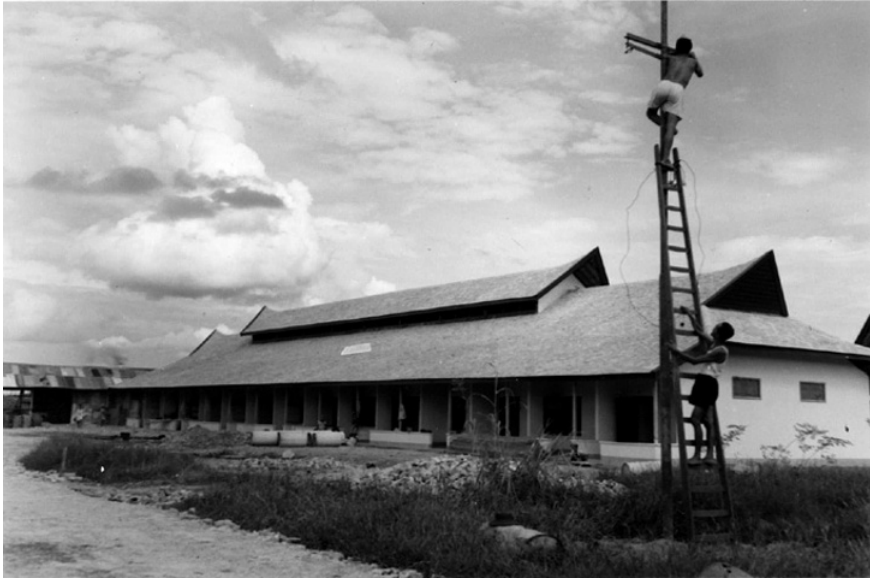
FIGURE 12.3 Barracks with vernacular-style roof for BPM labourers, 1930
