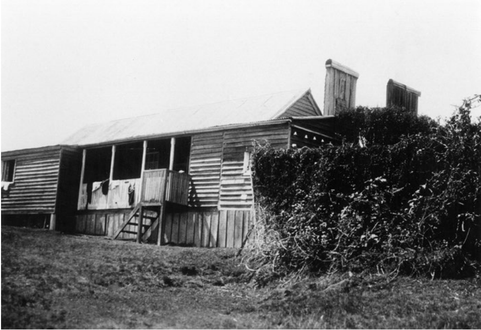
Figure 33: The Hamon's cottage and telephone office c. 1930. The extended house also served as the original guest house.
