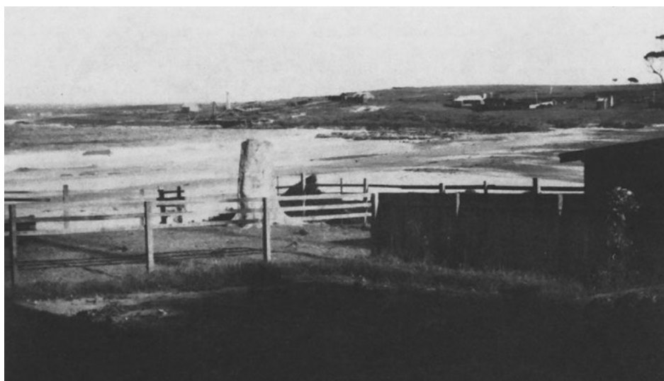
Figure 37: Bawley Point c. 1927, after the mill fire.
