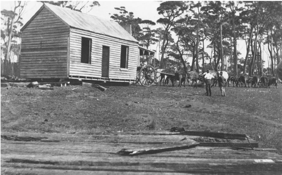
Figure 40: Moving two rooms of one of the mill cottages at Bawley Point to a site near the north end of Bawley Point Beach. These rooms became the centre of the cottage lived in by Broda and Henry Reynolds, and presently owned by Pat Johnson. Henry Reynolds (left) and Charlie Clark (bullock driver), c. 1925.
