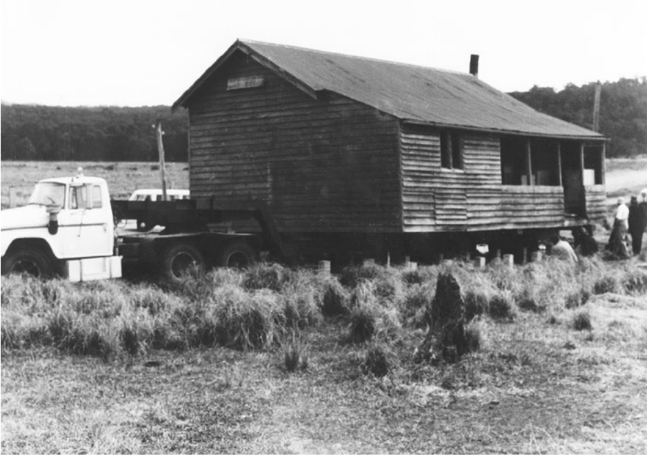
Figure 22: Kioloa school house being relocated closer to The Avenue.
