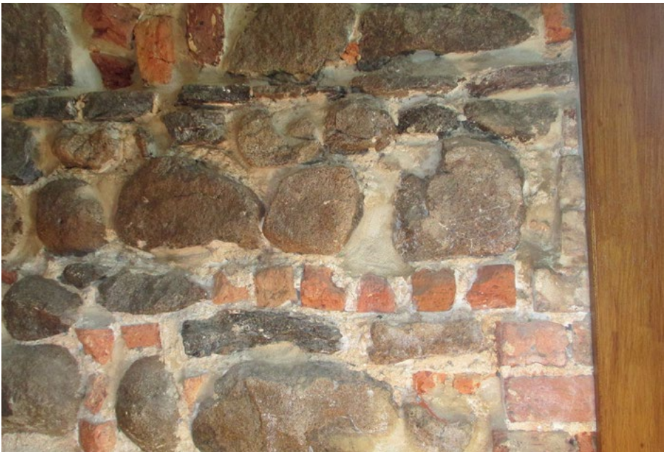
Figure 8: Wall construction, Murramarang House.
