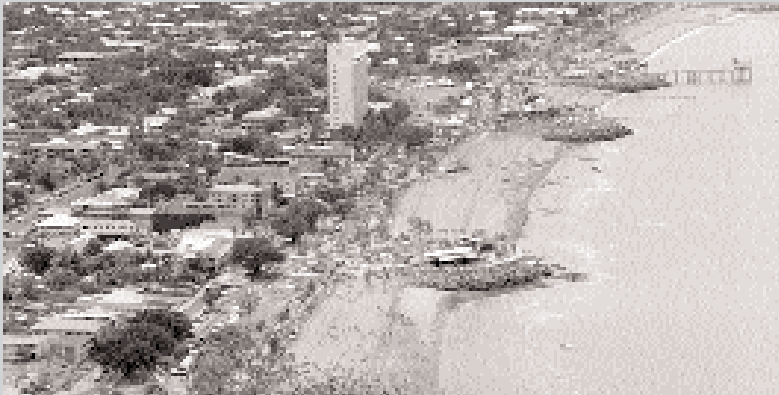
Figure 4.6 The Townsville foreshore beach after reconstruction
