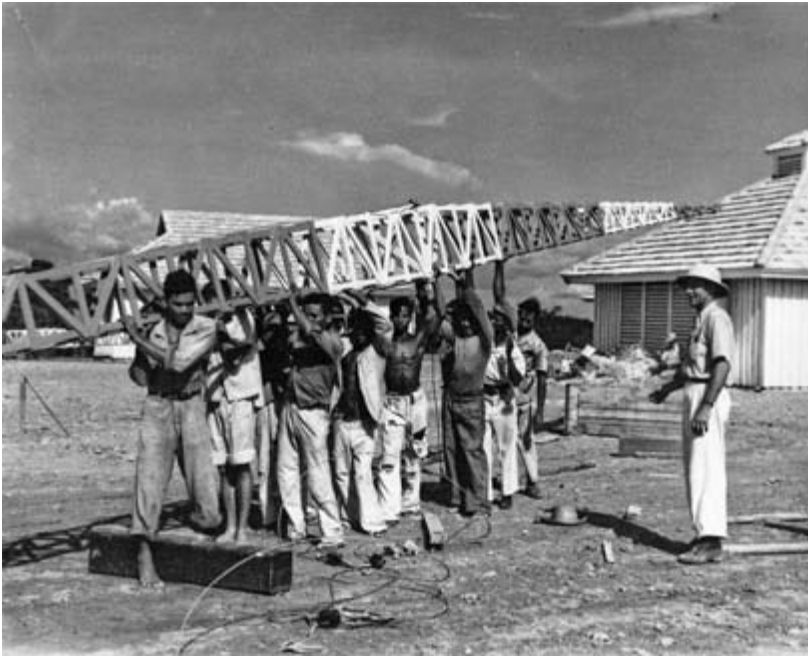
Figure 5.6 Migrants erecting radio tower at newly constructed airport in Manaus, February 1944. Source: National Archives.
