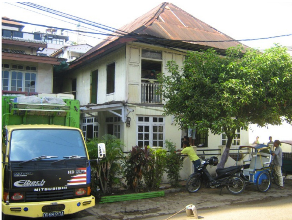
Figure 10.1 Unusu Daeng Remba's house in Jalan Maipa, Makassar, shortly before its demolition on 3 November 2011
