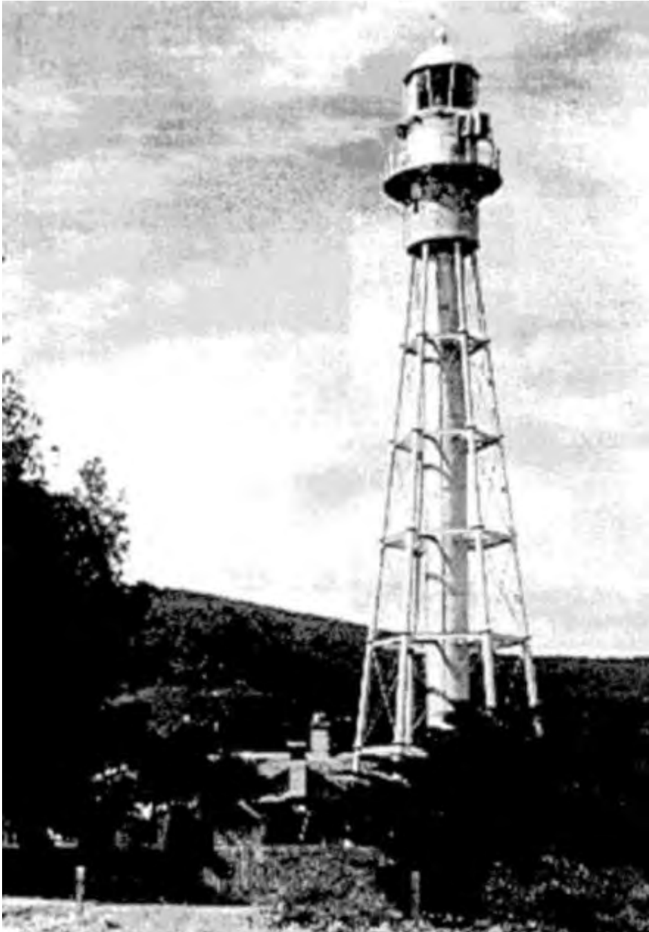
Fig 43. 'South Channel Lighthouse', perspective showing that the lighthouse was constructed adjacent to, not behind, the keepers' cottages
