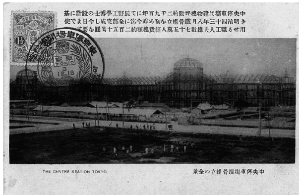
Figure 8: “The Centre Station Tokyo” under construction, Picture postcard, postmark Showa 3 (1914)
