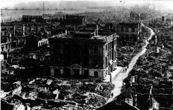
Figure 9: Tokyo after the Great Kanto Earthquake in 1923, view from the top of the Imperial Hotel by J. H. Messervey
