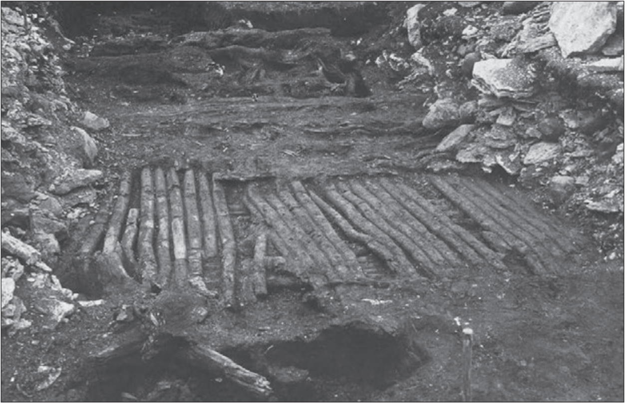
Fig. 17. Limestone rampart with log raft foundation at the fort at Kuusalu (photo: E. Saadre, 1936, AI).
