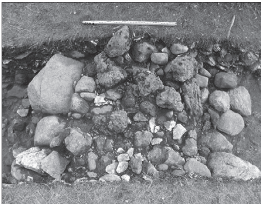
Fig. 34. Construction of the stone wall in Lipa (photo: V. Lang).
