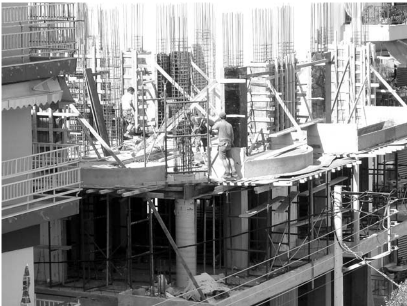
Photo 7 Albanian migrants working in construction, Thessaloniki
