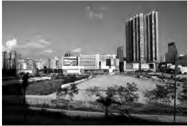
Figure 9.6 Elements Mall: an Atrium leading to the Airport Express Rail
