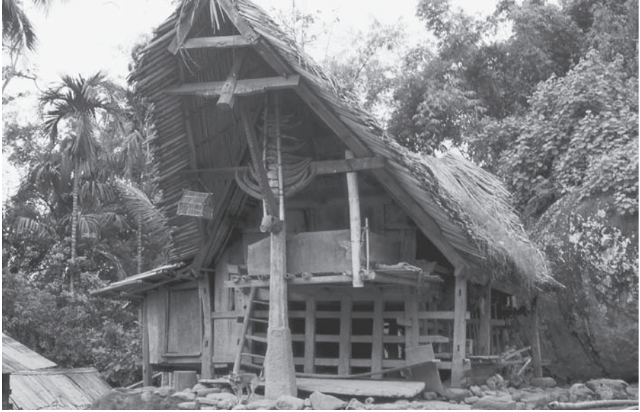
An old tongkonan in the hamlet of Kata, on the hillside above Buttang, 1994. Older houses were comparatively small and lacked the exaggerated projection and curve of the roof which is now fashionable.
