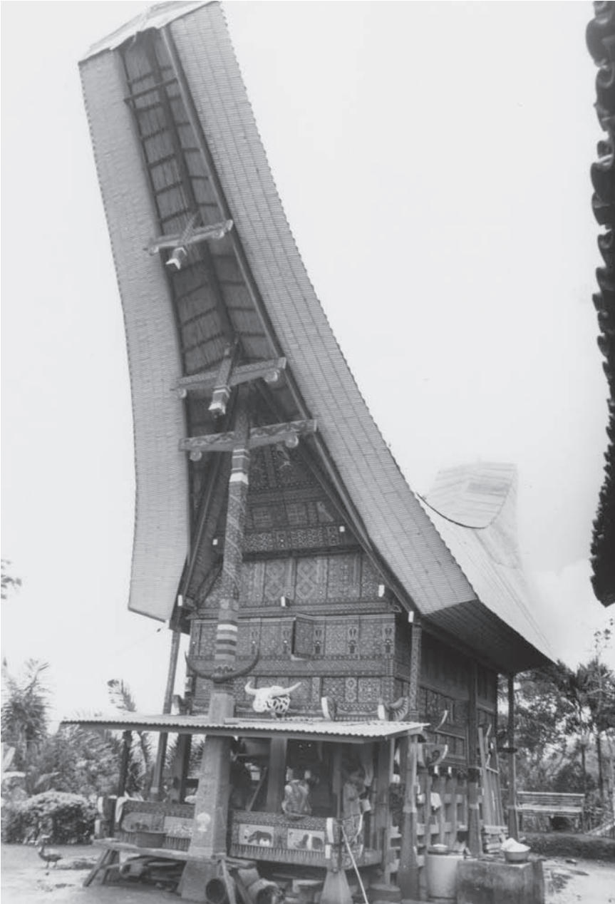
A recently rebuilt tongkonan in Menduruk showing the dramatically projecting eaves typical of newer constructions, and a style of carving influenced by carpenters from Rantepao, 1999
