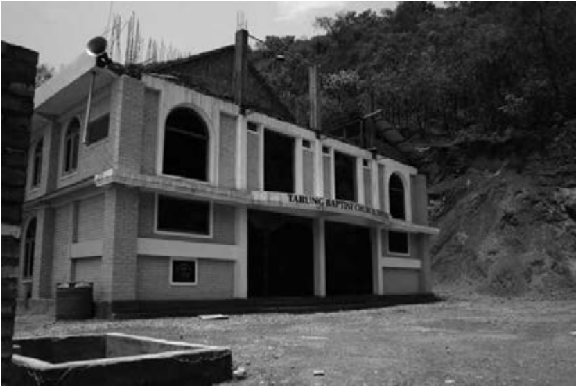
Image 6.2 Baptist church under construction, Langol
