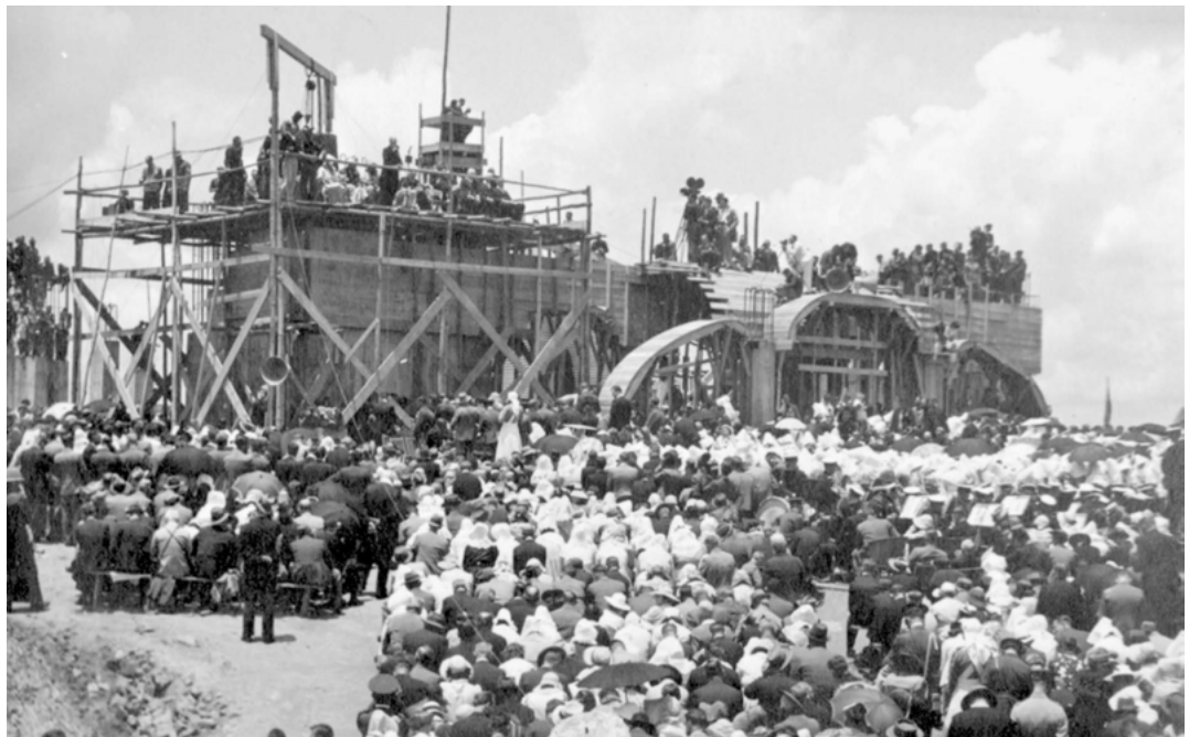
Figure 30: Laying of the Voortrekker Monument foundation stone on 16 December 1938 (photo courtesy of Unisa Archives)
