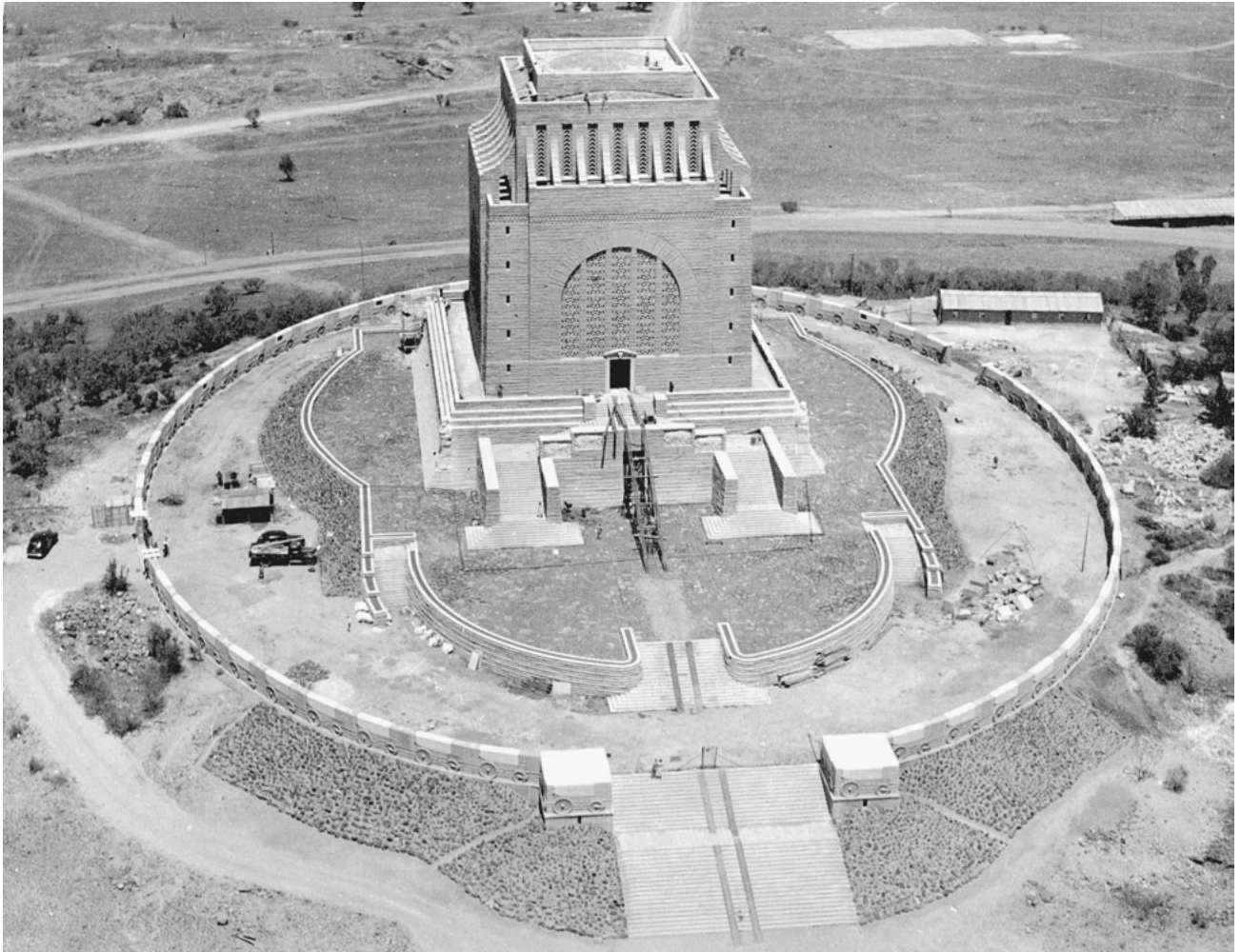
Aerial view of Voortrekker Monument in 1949: building site with ramps for transporting the completed marble panels into the Hall of Heroes (photo courtesy of Unisa Archives, Van Schaik album)
