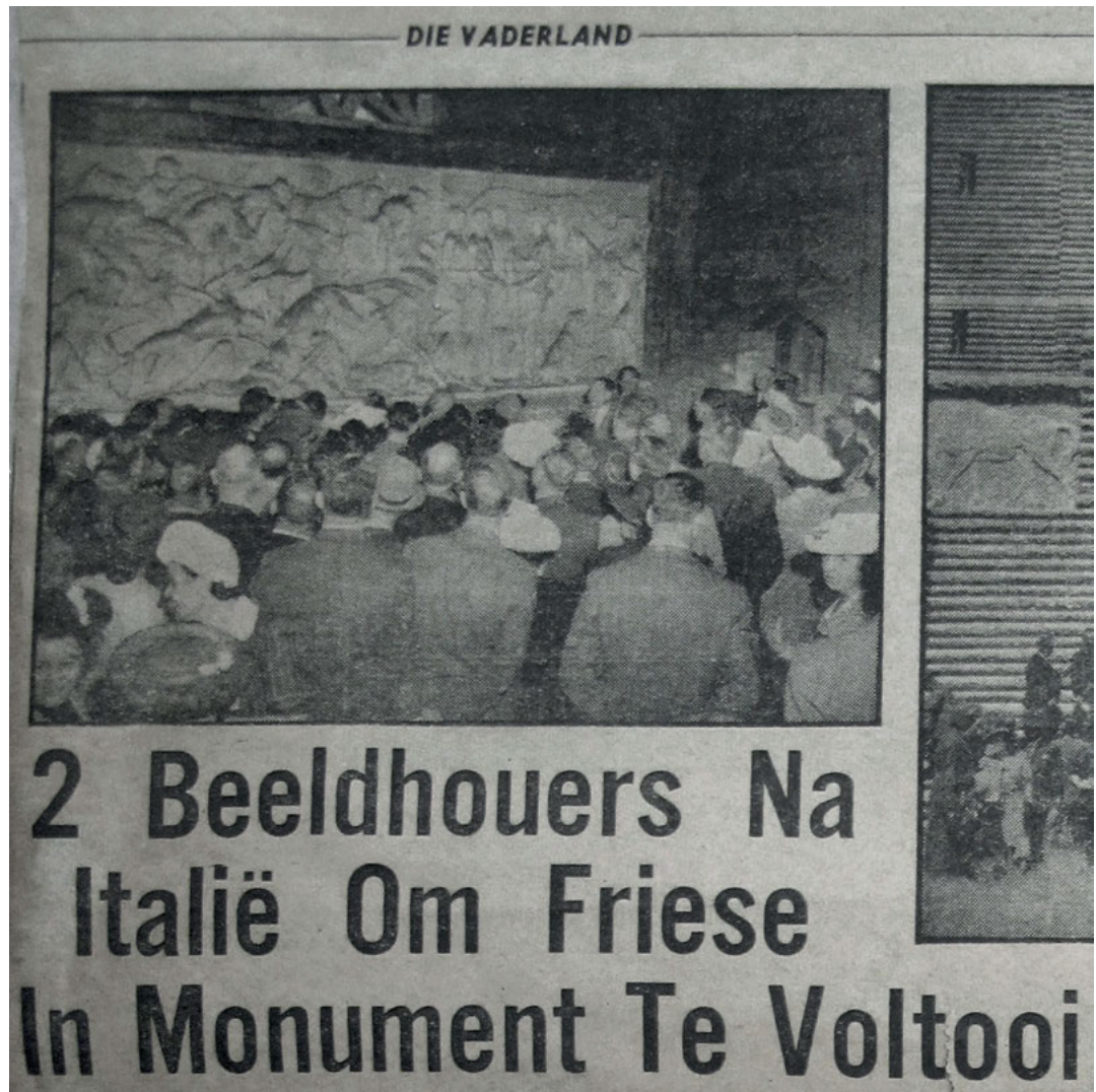
Figure 189: Plaster casts of Kapain and Negotiation in situ in Monument. Corner panel of Blydevooruitsig already removed ( Die Vaderland 10.9.1947; courtesy of UP Archives, Moerdyk files)
