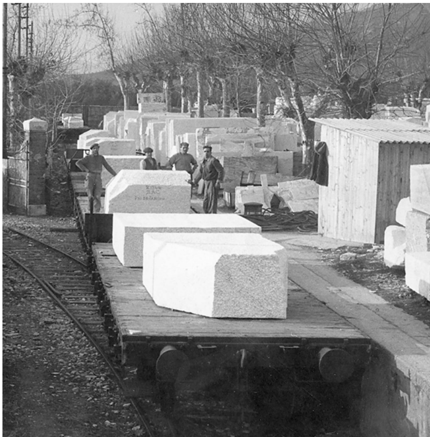
Figure 201: Marble panels ready for transportation. 1948 (courtesy of UP Archives, Postma files; photo N. Lughetti, Forte dei Marmi)
