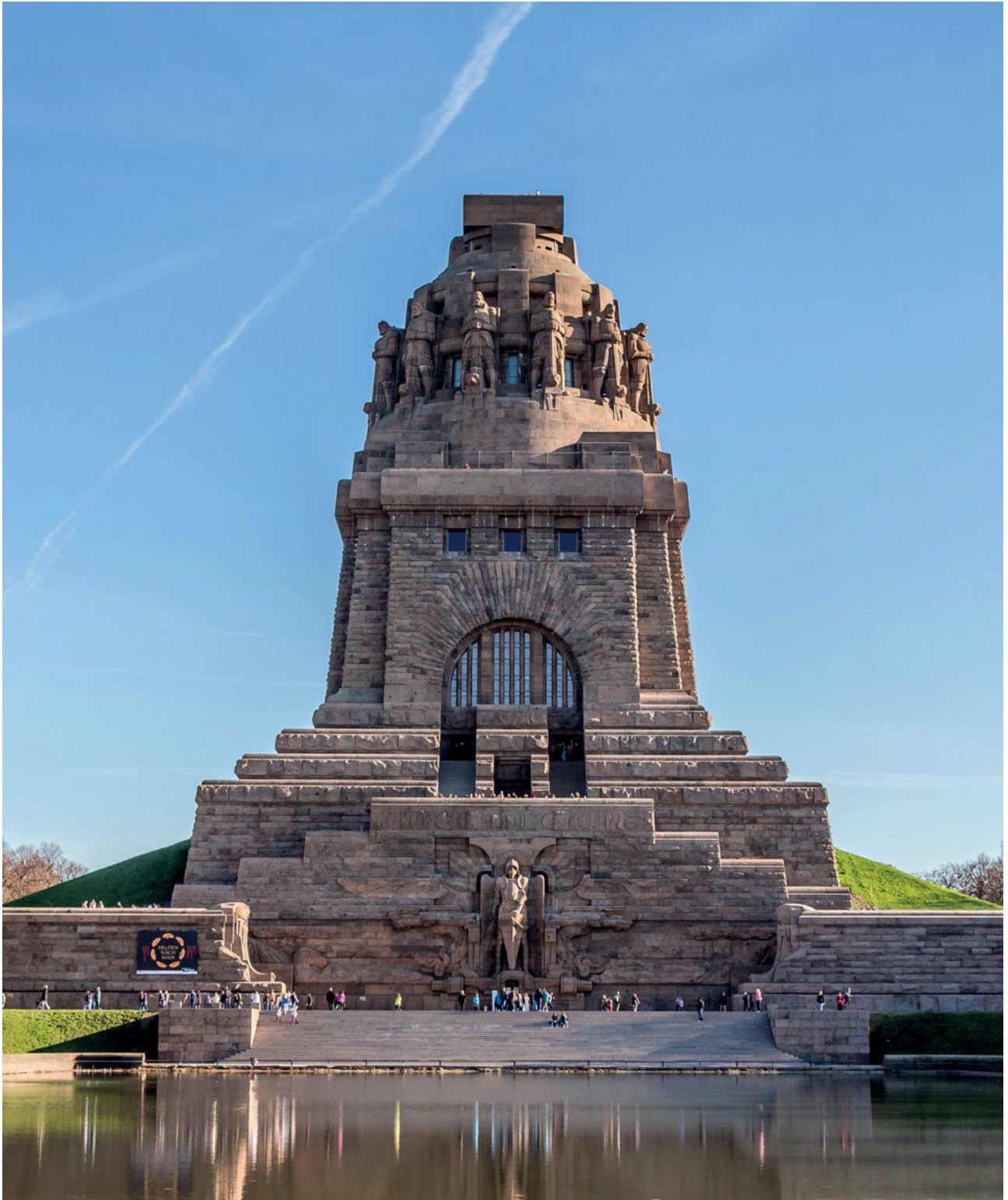
Figure 76: Bruno Schmitz et al. Völkerschlachtdenkmal, Leipzig. 1913. Steel and concrete with granite facing, h. 91 m, plinth 70 × 80 m (photo courtesy of Alamy GGD80)
