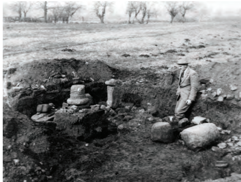
Fig 2.14 Photograph of the excavations just inside the North Gate by Barber et al in 1924 (G34/3). Viewed from the south east. Unknown photographer. Reproduced by courtesy of Sir Andrew Lawson-Tancred
