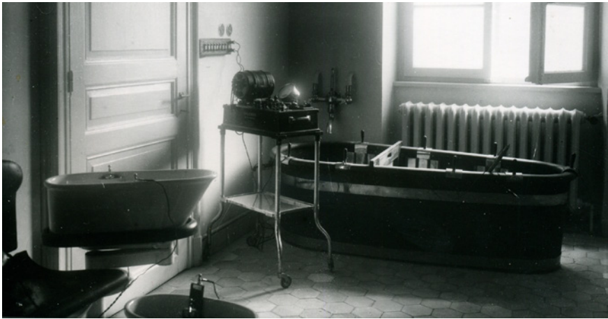
FIGURE 0.8 Hydrotherapy installation—ionization by electrolysis (1923).
