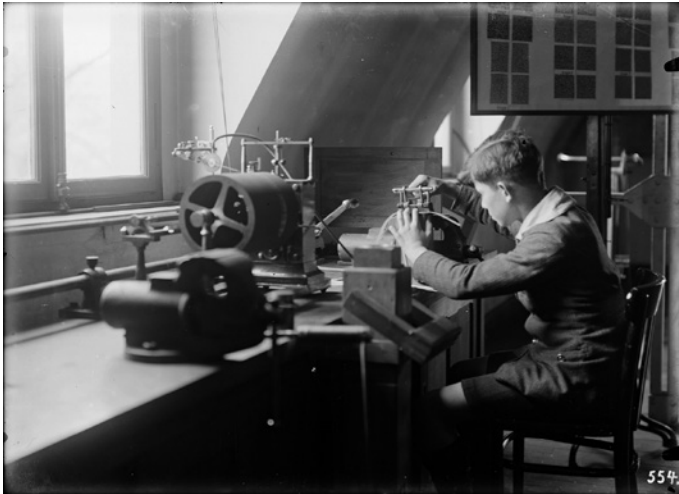
FIGURE 4.1 Perforating test in the laboratory of the Institut Emile Metz. © INSTITUT EMILE METZ. CNA COLLECTION.
