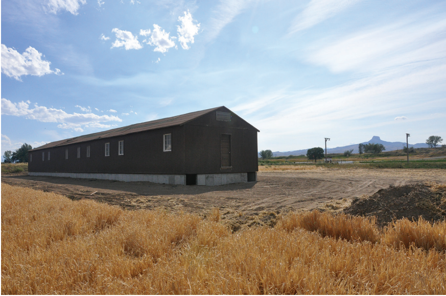
FIGURE 10 Reassembled barrack on the site of the Heart Mountain Relocation Center, 8.15. PHOTO COURTESY OF BRIAN LIESINGER, HEART MOUNTAIN INTERPRETIVE CENTER.
