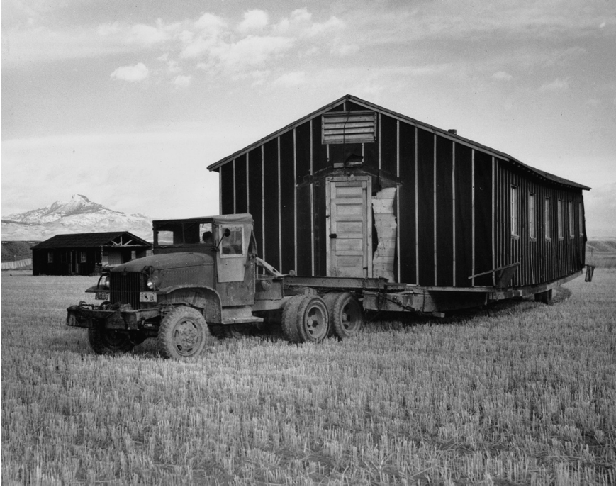
FIGURE 4 A section of William A. Cannon's barrack, on the truck. SHOSHONE IRRIGATION DISTRICT.
