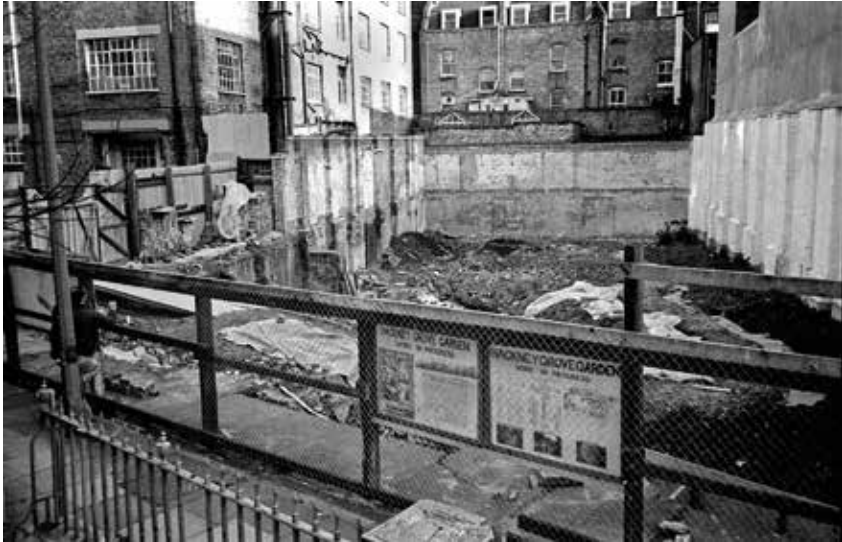
Figure 7.9. Hackney Grove Gardens 'Work in Progress', Jan. 1983. Photo: Alan Denney via flickr.
