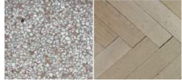
Fig. 6. Mosaic and wooden floor structure.
