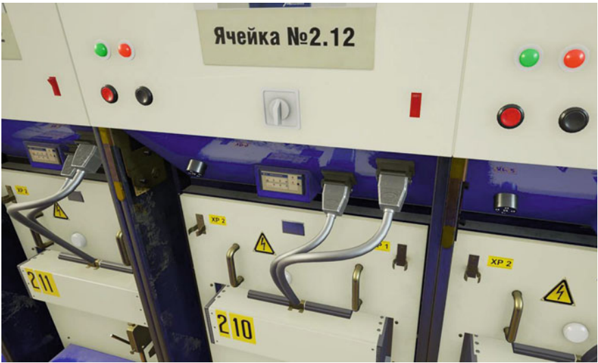
Fig. 19.10 Detailed 3-D functional model of 10 kV circuit-breaker
