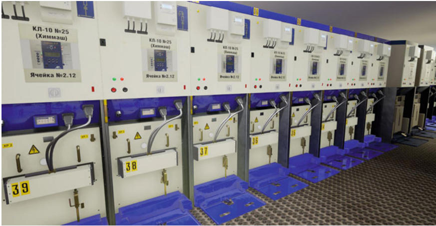
Fig. 19.9 3-D model of 10 kV indoor switchgear group
