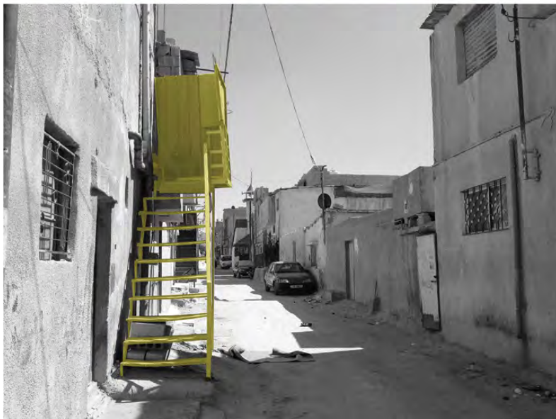
Figure 25.6 As the horizontal planes became saturated with cement, refugees devised another ‘architectural element’ in the form of external stairs to serve as a facilitator to vertical expansion. © Samar Maqusi.
