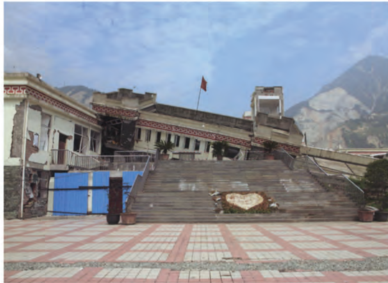
◀ Xuankou High School after the earthquake
