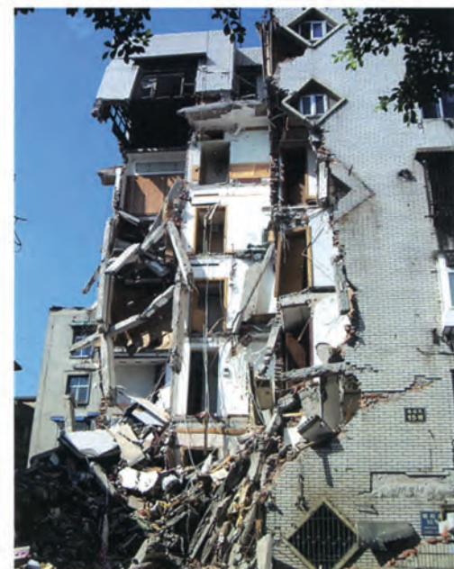
▲ Collapsed building in the town of Guangji
