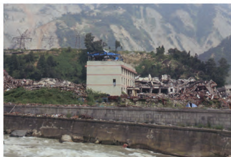
A building destroyed by the earthquake
