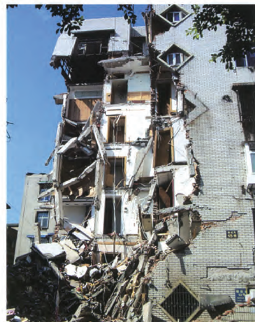
▲ Collapsed building in the town of Guangji
