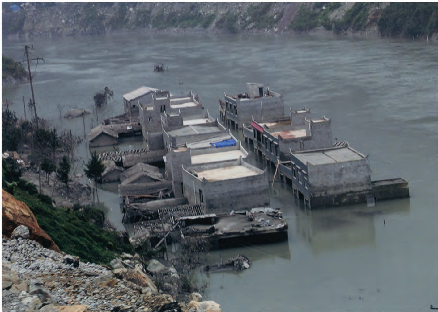
▲ This photo shows construction sites that were submerged because of water levels rising and the Minjiang River becoming narrower because of landslides and collapses.
