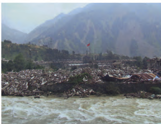
Yingxiu Primary School after the earthquake
