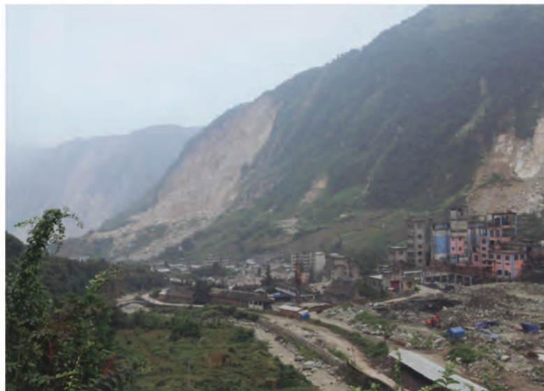
◀ The town of Xuankou after the earthquake
