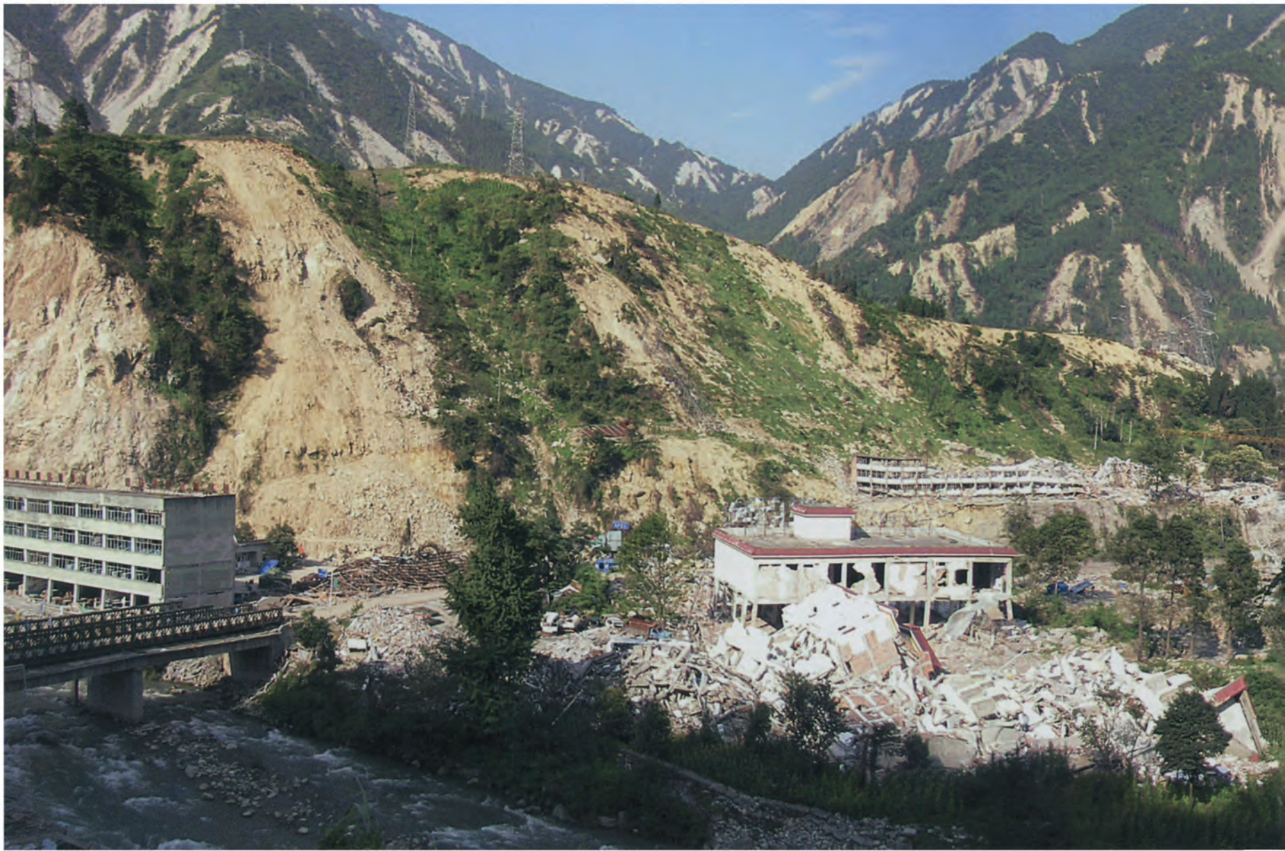
A photo of the town of Yingxiu after the earthquake
