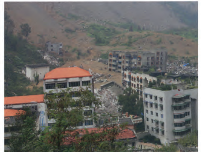
Administration building of Beichuan County
