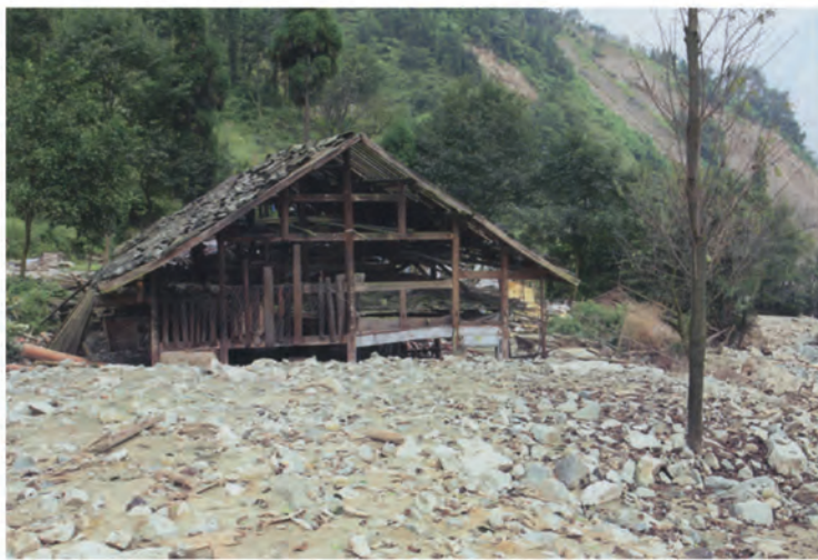
A building destroyed by debris flow
