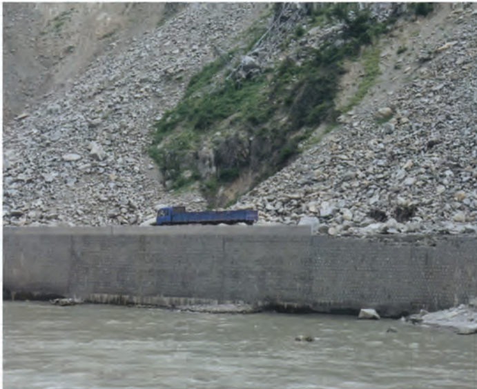
Photograph of earthquake debris flood.
