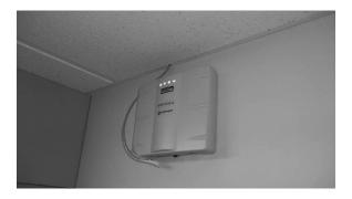
Figure 9.3 Example of poor cable installation.
