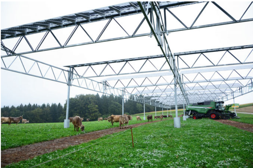
Photo 8.1 Multiple land use by an agrophotovoltaic plant that enables solar power and crops to be harvested simultaneously from one plot (source ISE Fraunhofer)
