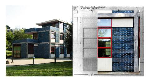
Fig. 4 – From the left, view of one of the 4 wings of the building, comparison between the photo-rectification and the executive drawing of the type c module.
