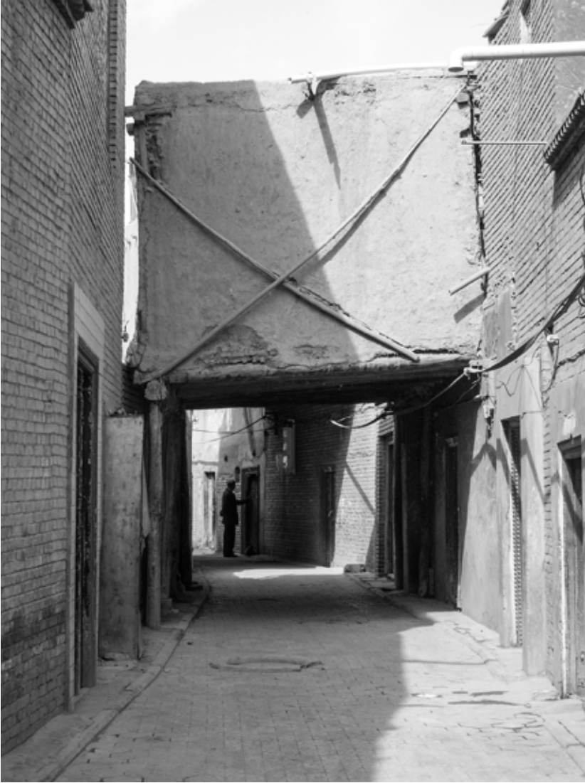
Figure 13: A typical section of old Kashgar, before the renewal (picture by the author, 2013)
