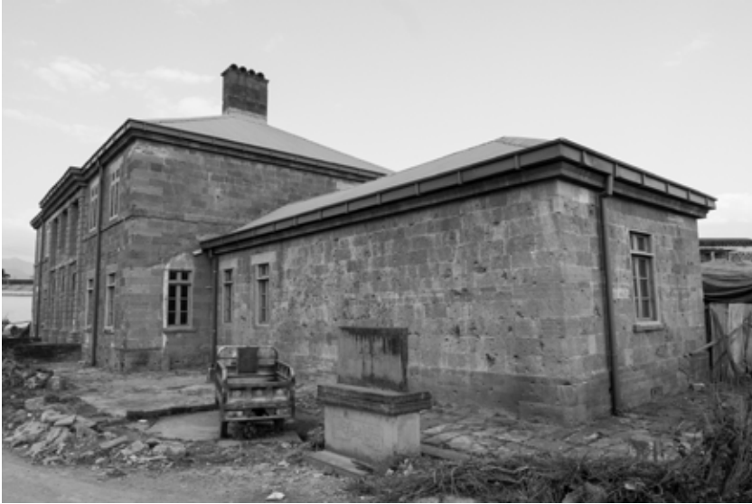
Figure 6: Former British consulate in Tengchong (picture by the author, 2016)
