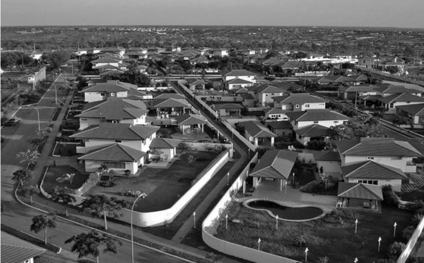
Figure 7.3 Private Condominium Atlantico do Sul in Belas Municipality, Luanda
