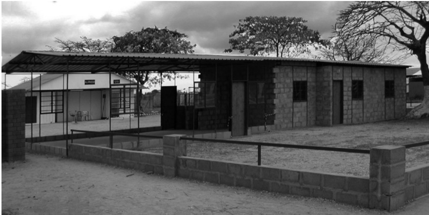
Figure 7.6 Incremental (Upgradeable) House in Zango
