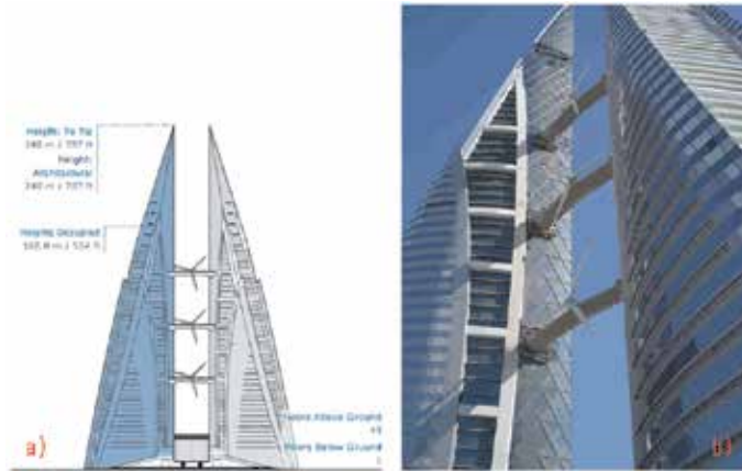
Figure 2. Wind turbines integrated in between the Bahrain world trade Center towers; elevation view (a) and a general view from the pedestrian level (b) [7].
