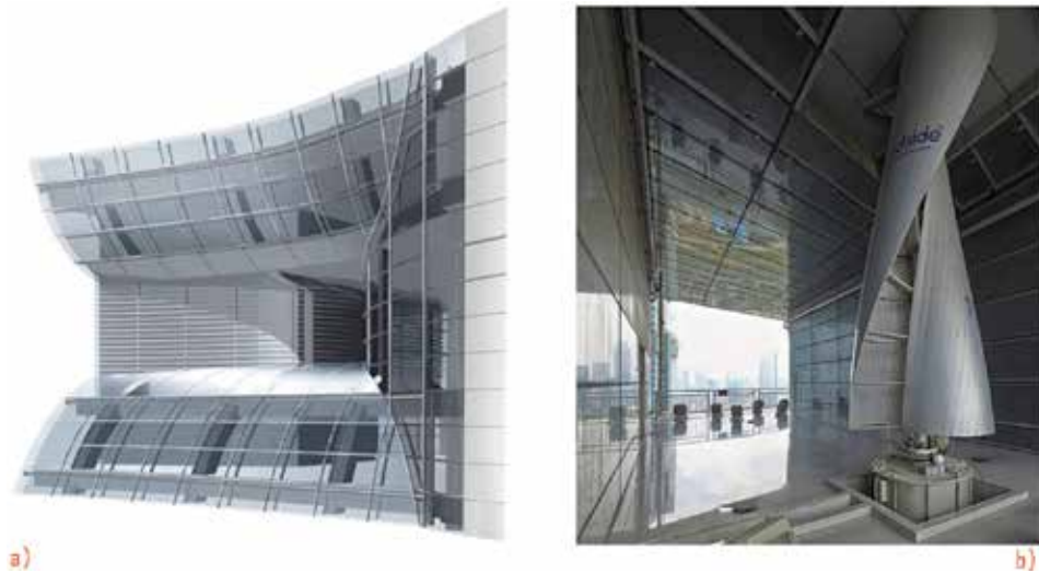
Figure 10. Pearl River tower; aerodynamic configuration on the facade (a) and the detailed view of the helix-shaped vertical-axis wind turbine (b) © SOM.
