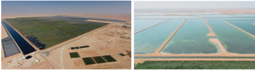
Figure 6.5 Case study 4 – Nimir Water Treatment Plant (Oman). (Pictures reprinted with permission from Bauer Nimir LLC)
