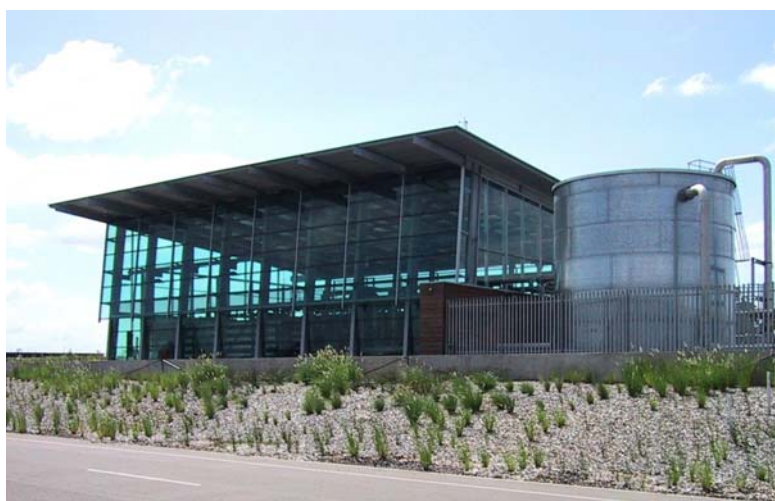
Figure 11.2 Homebush Bay Water Recycling Plant (Photograph courtesy of Sydney Olympic Park Authority).
