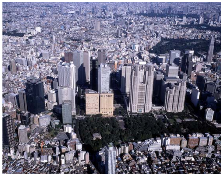
Figure 12.4 Views of the high-rise buildings in the Shinjuku area in Tokyo supplied with recycled water for toilet flushing.
