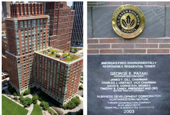
Figure 13.1 The Solaire – America's first high-rise residential green building.
