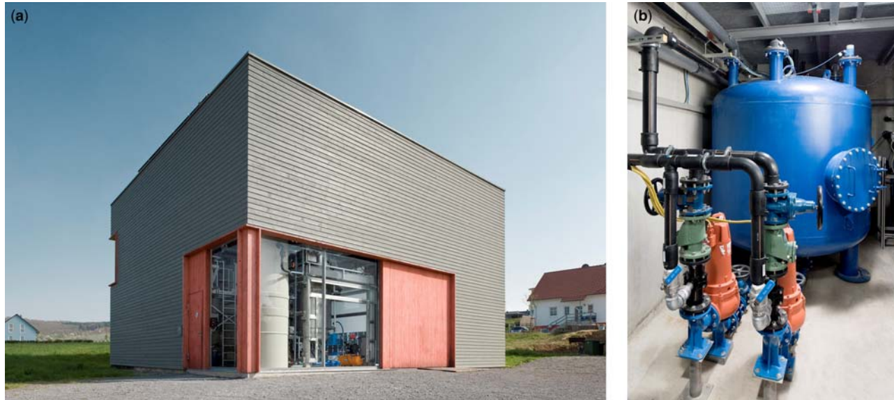
Figure 7.1 Photographs of the “Wasserhaus” in Knittlingen and the vacuum station in the basement.
