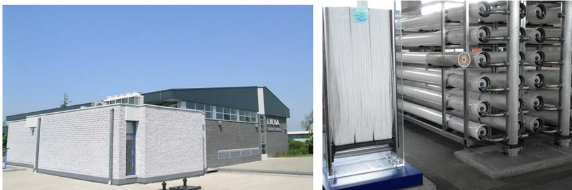
Figure 26.1 General view of the Torreele recycling facility and the membranes of ultrafiltration and reverse osmosis.
