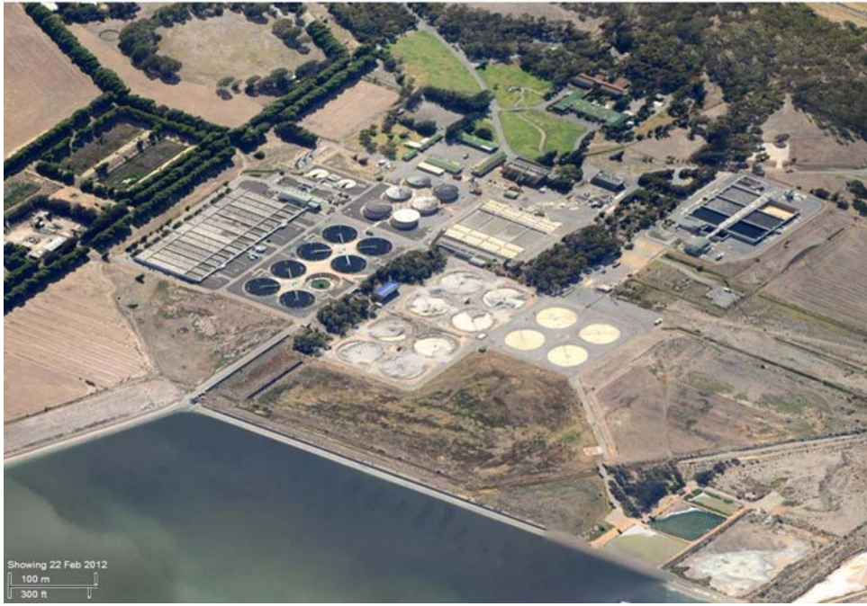
Views of the Bolivar water recycling plant.
