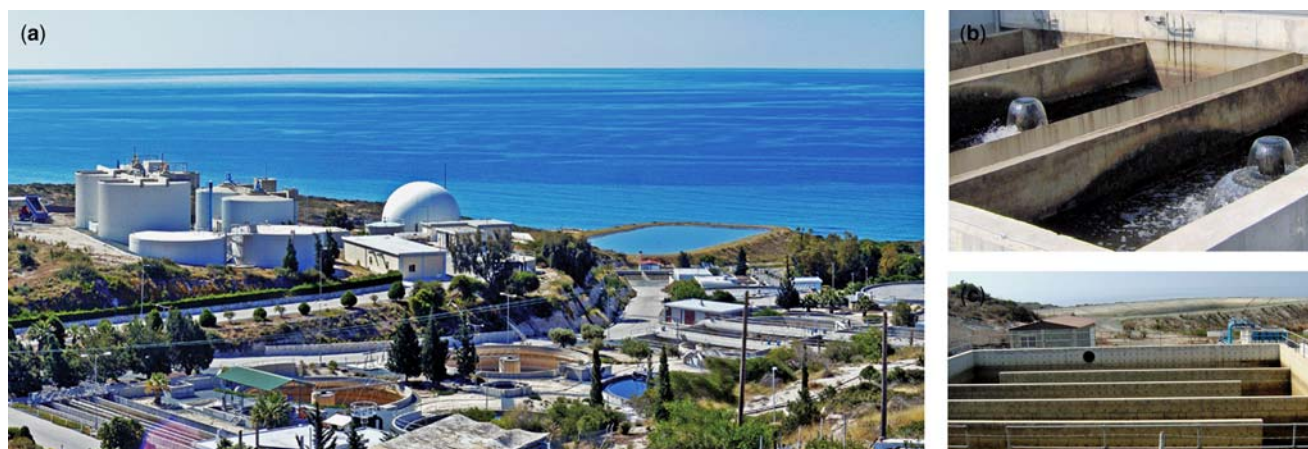
Figure 5.2 (a) A general view of the biological WWTP of Limassol (b) the tertiary treatment stage of sand filtration and (c) chlorination (the storage tank can be also seen at the back).
