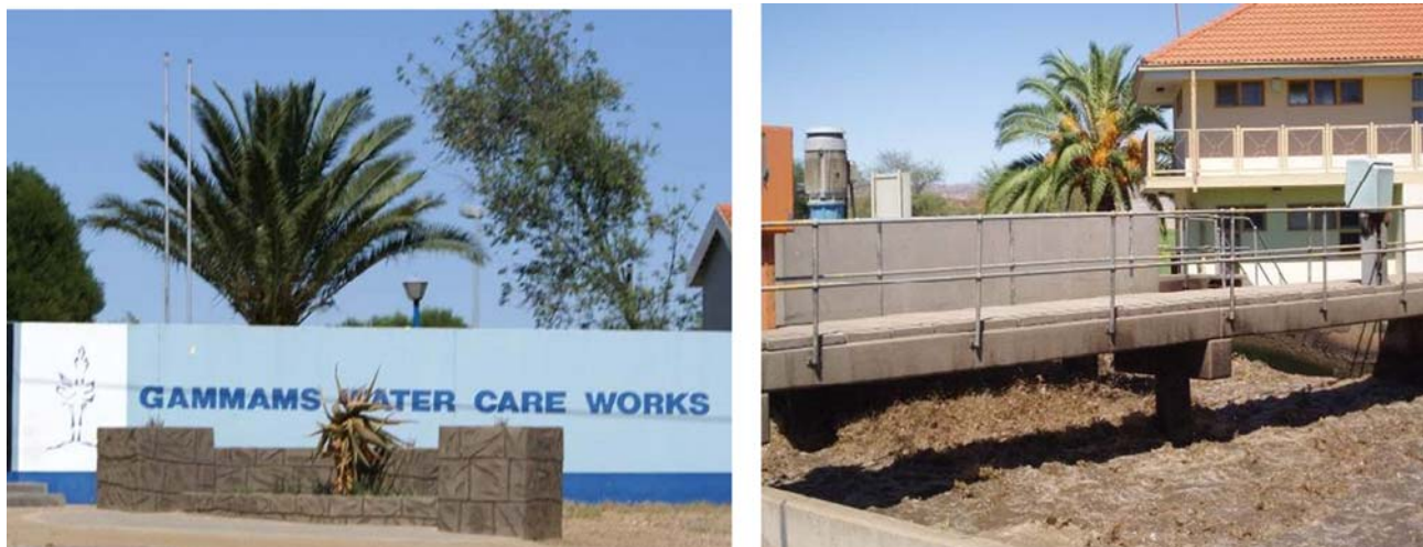
Figure 29.3 View of conventional biological wastewater treatment at the Gammams Water Care Works.
