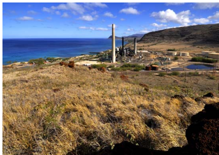
View of a large power plant in Honolulu.
