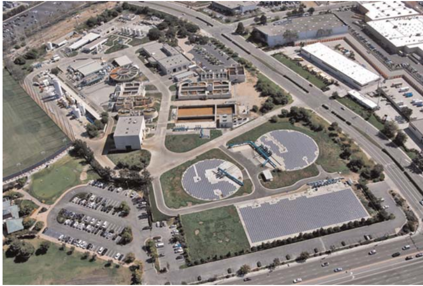
Figure 2.6 Aerial view of the Edward C. Little Water Recycling Facility in West Basin with solar panels.
