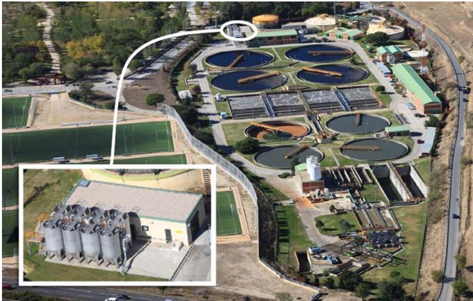
Panoramic view of one of the tertiary treatment process in the Community of Madrid.
