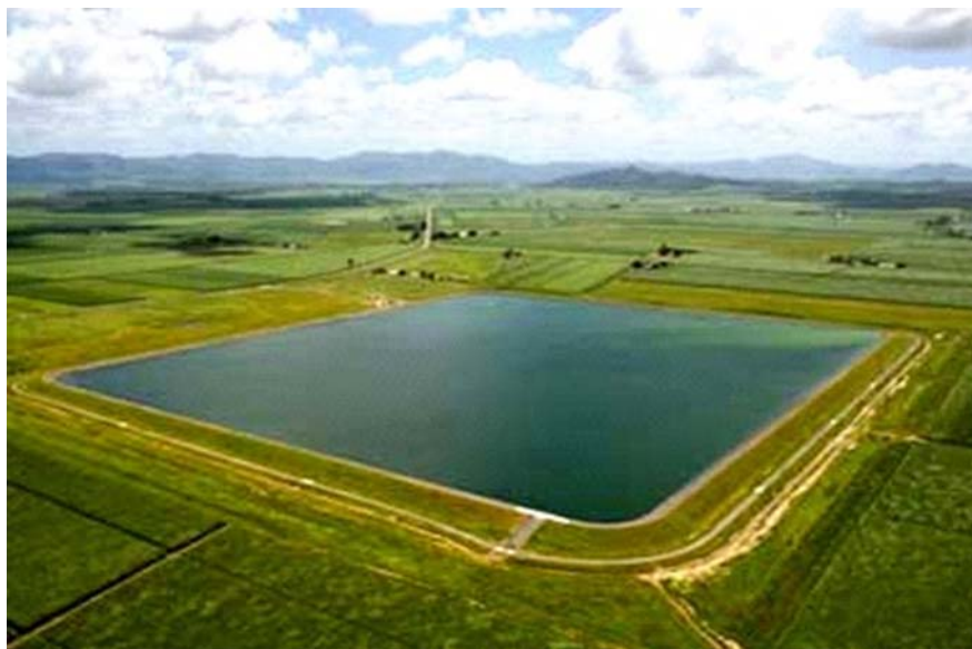
Figure 17.2 Recycled water storage, Mackay water recycling scheme (Photograph courtesy of Smart Water Australia, Canberra).
