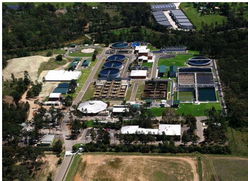
Figure 11.3 Rouse Hill Water Recycling Plant (Photograph courtesy of Sydney Water).
