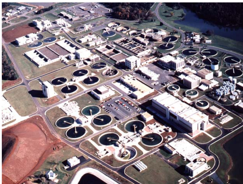
Figure 27.3 Aerial photo of a portion of the 204,400 m 3 /d (54 MGD) UOSA water reclamation plant known as the Millard H. Robbins, Jr. Water Reclamation Facility.
