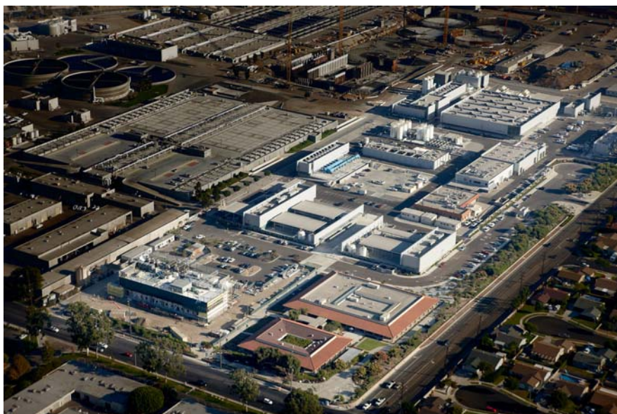
Figure 25.11 Aerial view of the Advanced Water Purification Facility (Photo credit: Larry Mack).
