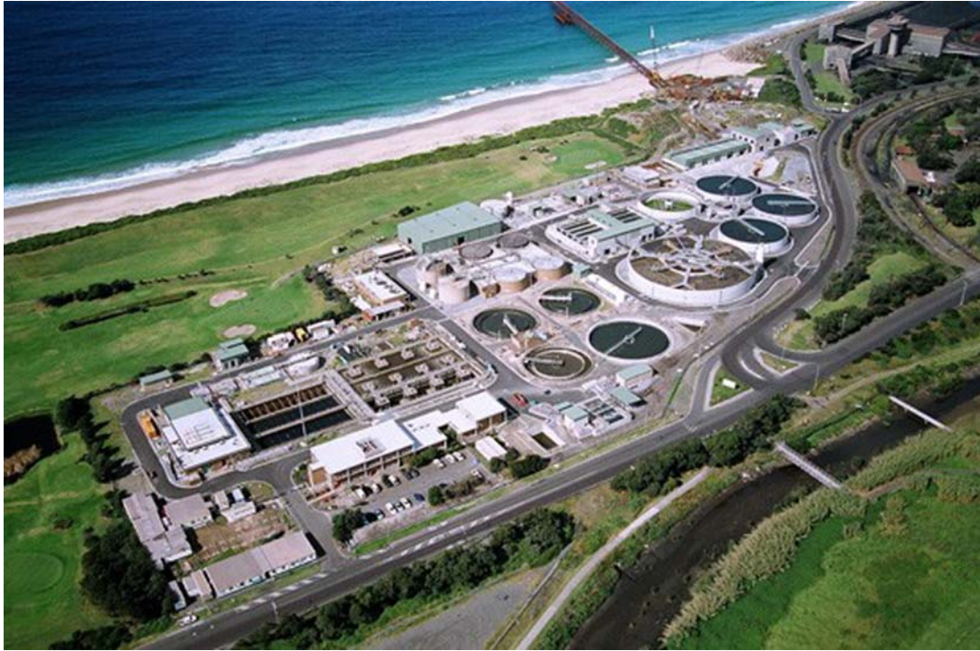
View of the Wollongong Sewage Treatment Plant in Sydney (Photograph courtesy of Sydney Water).
