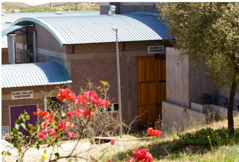
Views of the New Goreangab Plant in Windhoek.
