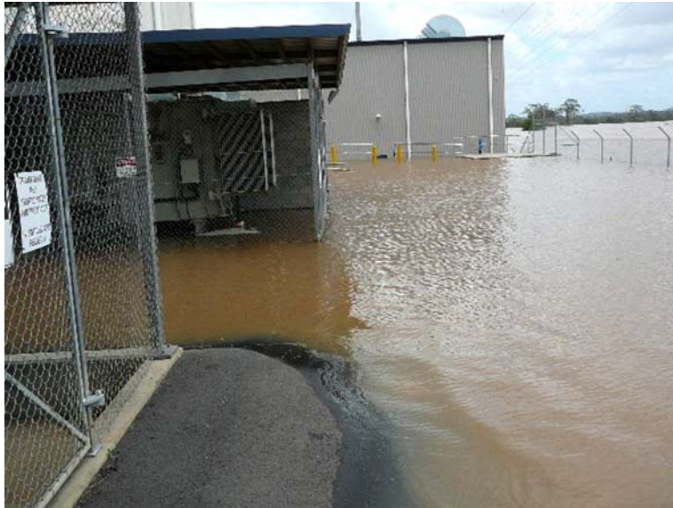
Figure 28.6 Bundamba AWTP during the 2011 Brisbane flood.
