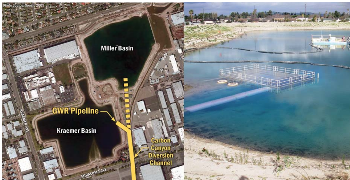
Figure 25.10 Views of Kramer Basin recharge facilities and Miller basin, inlet structure and the district's cleaning machine.
