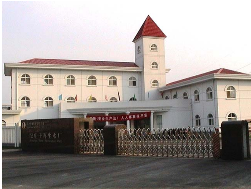
View of the Ji Zhuangzi water reclamation plant.
