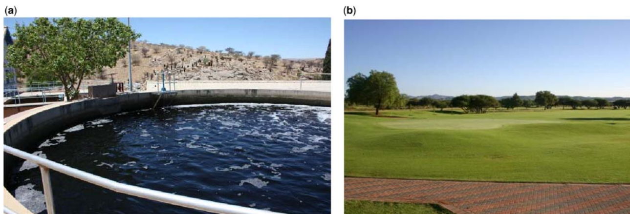
Figure 29.5 View of the Old Goreangab Water Reclamation Plant (a) and the golf course of the Windhoek Country Club (b).
