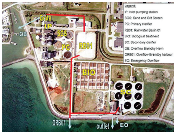
Figure 6.24: Aerial view of Avedøre WWTP.
