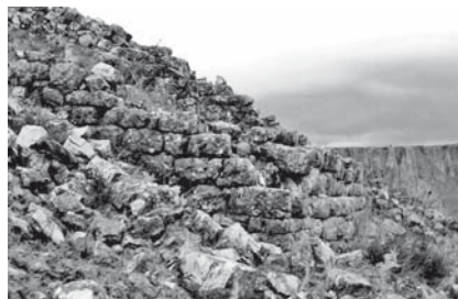
Fig. 73: Fortification on the summit of Mt. Nitai: remains of one of the wall towers
