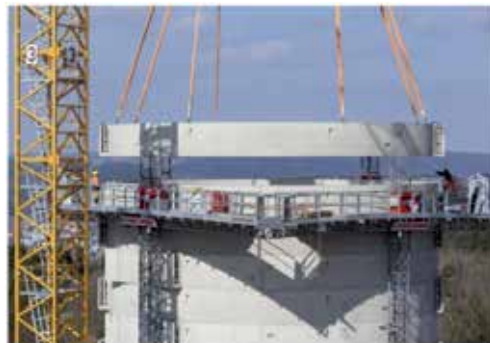
Figure 8. Hybrid tower on the concrete foundation (Credit: Liebherr Plant Ehingen GmbH).
