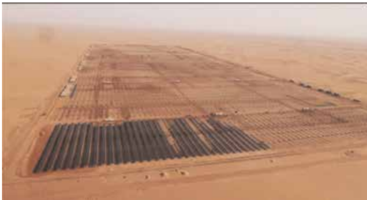
Figure 4. Aerial view of under construction Benban PV power plant in Egypt [14].
