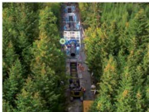
Figure 12. The operation of the PiPECrawler in Gaildorf (Credit: Max Bögl).
