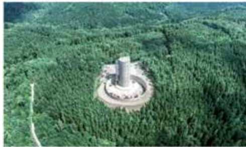
Figure 10. Lower part of the tower including the short-term storage (Credit: Max Bögl).
