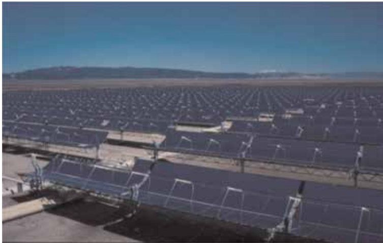
Figure 7. Largest parabolic-trough concentrated solar system.
