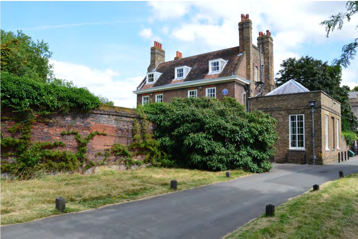
Figure 1.4: Wilderness House . Brown is the only 'landscape architect' to be recognised with a 'blue plaque' as a commemorative historical marker. It is on Wilderness House, his former residence at Hampton Court Palace. Photo copyright Jan Woudstra, 2016, CC BY-NC 4.0.
