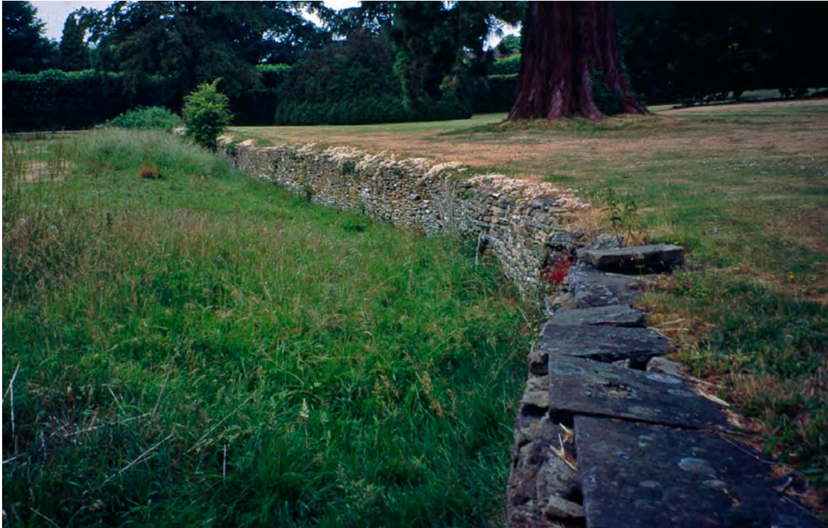
Figure 8.6: Richmond's serpentine ha-ha defining the pleasure ground he made at Badminton House. Photo copyright David Brown, CC BY-NC 4.0.
