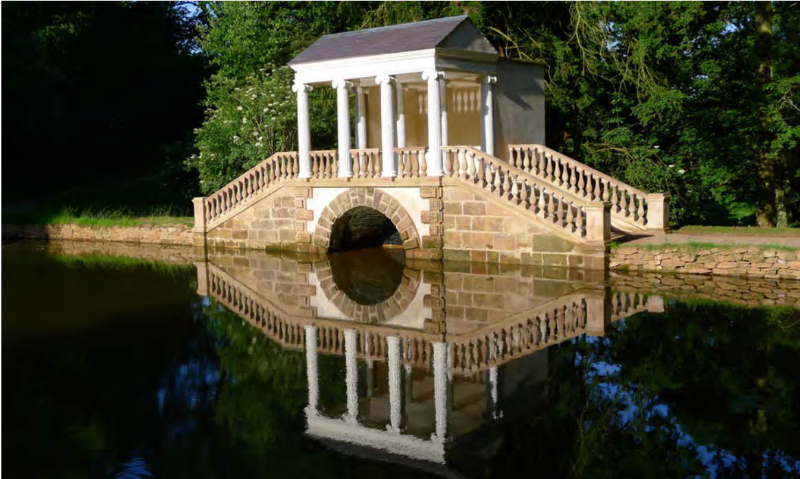
Figure 13.2: The restored Hagley Bridge today, at Hagley Hall. Photo copyright Laurent Châtel, CC BY-NC 4.0.
