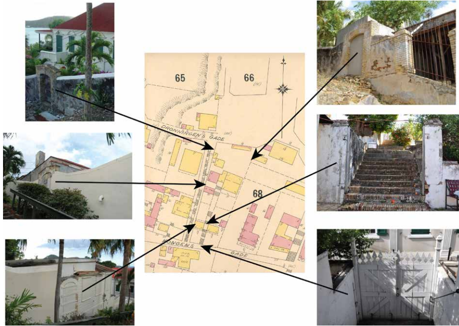
Figure 4 19 th century gates at the Magens House with gateways located on 1893 Goad Insurance Map.
