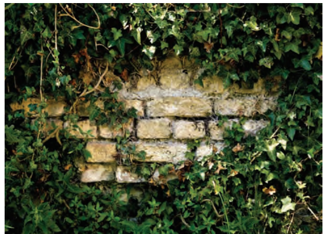
Fig. 11.13: Bricks from the east face of the Bulwark rampart (P. W. © English Heritage DP068603)
