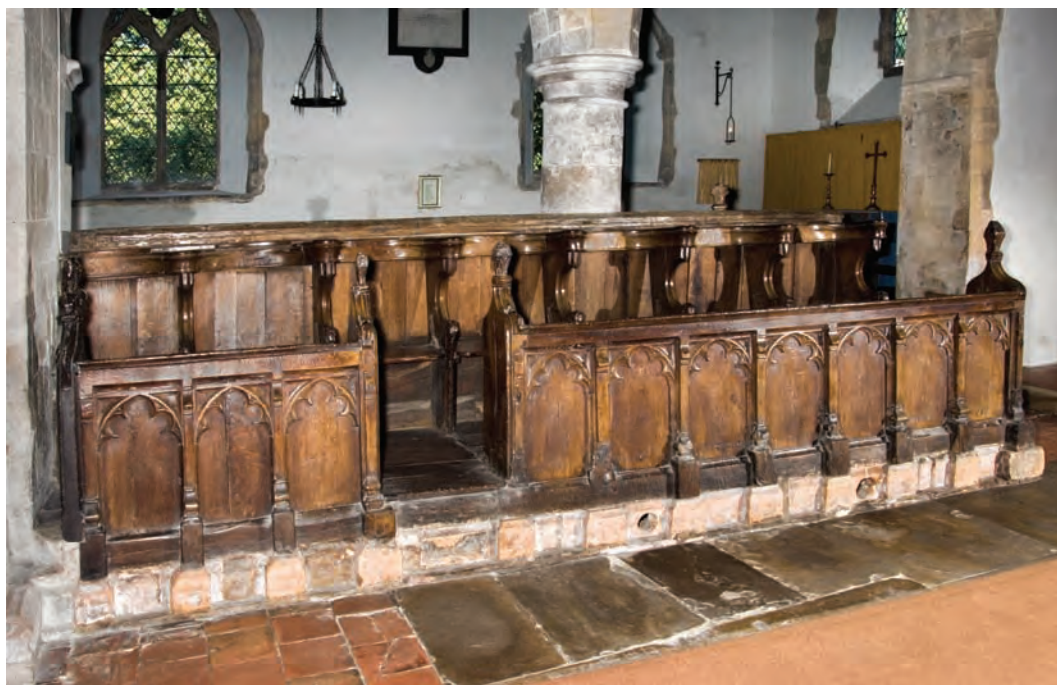
Fig. 13.6: St Clement's church, choir stalls with holes for acoustic jars below (P. W. © English Heritage DP044030)
