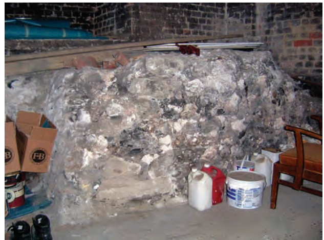
Fig. 11.16: The core of the town wall in the cellar of The Bell Hotel (K. P.)
