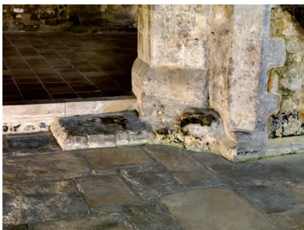
Fig. 3.9: St Peter's church, pier base at north-west corner of tower, seen from north, suggesting porticus entry (P. W. © English Heritage DP032236)
