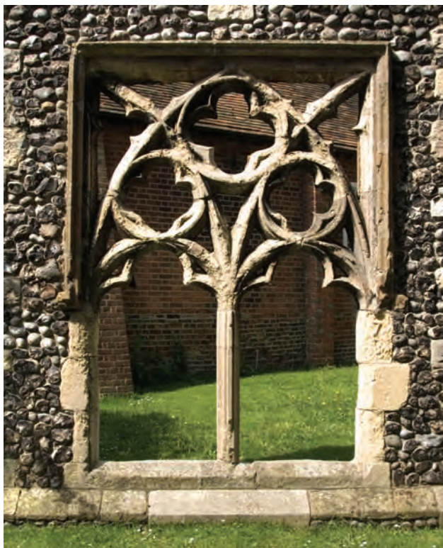
Fig. 13.9: Window from St Thomas's hospital, re-erected at the west end of St Peter's church (P. W. © English Heritage DP044012)
