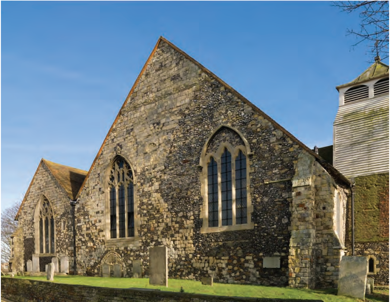
Fig. 6.6: St Mary's church, west end. The string course at the south end of the west wall and the lancet window in the north aisle indicate the widening of the south aisle in the thirteenth century (P. W. © English Heritage DP0322251)
