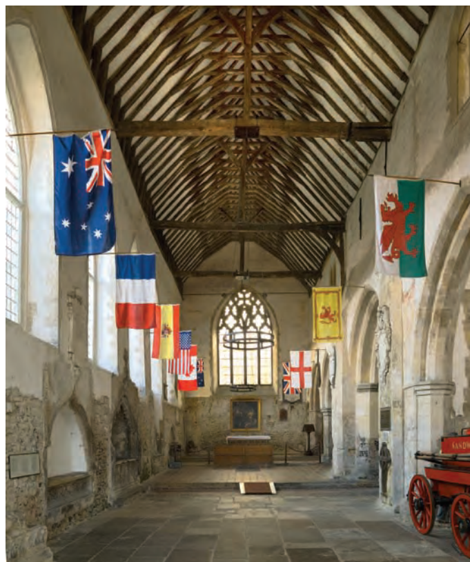
Fig. 6.16: St Peter's church, north aisle (P. W. © English Heritage DP032232)
