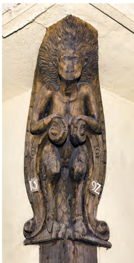
Fig. 16.17: The King's Arms Public House, 63, 65 Strand Street (House 91), caryatid carrying dragon beam (P. W. © English Heritage DP032252)
