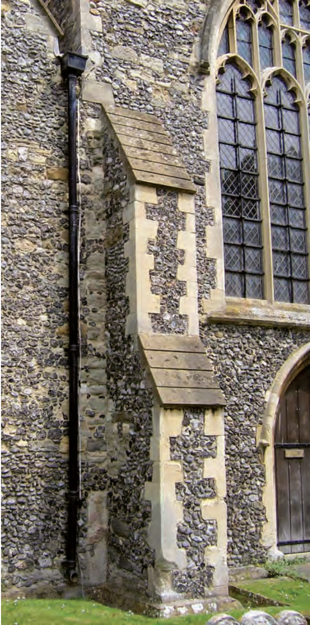
Fig. 3.4: St Clement's church, west wall, north side, straight joint of unaisled nave, with long Marquise stone at base to left of later buttress (S. P.)
