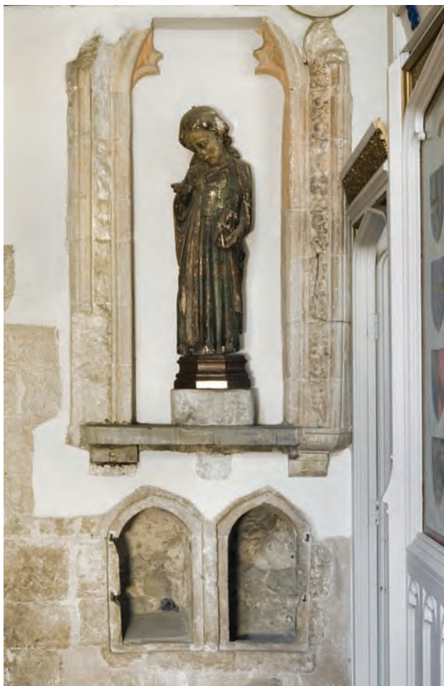
Fig. 13.5: St Clement's church, image niche and aumbries in St George's chapel (P. W. © English Heritage DP044052)
