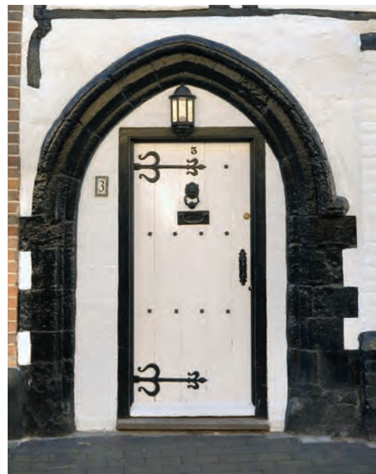
Fig. 7.17: Reset doorway at 3 Vicarage Lane (House 99) (P. W. © English Heritage DP032250)
