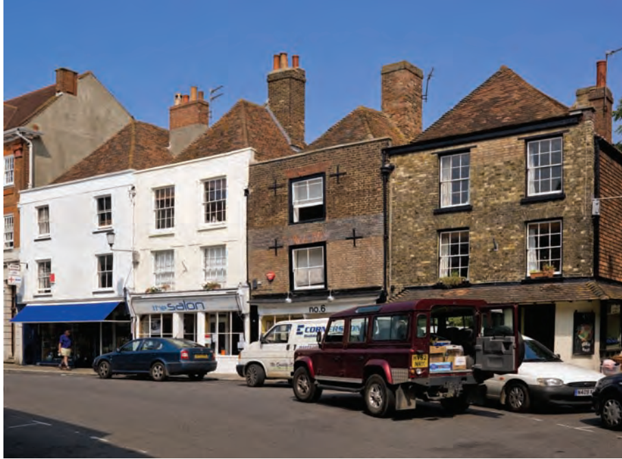
Fig. 12.13: 4, 6, 8, 10 Market Street (Houses 58, 57, 55, 53). Medieval houses in the former Fishmarket (P. W. © English Heritage DP068619)
