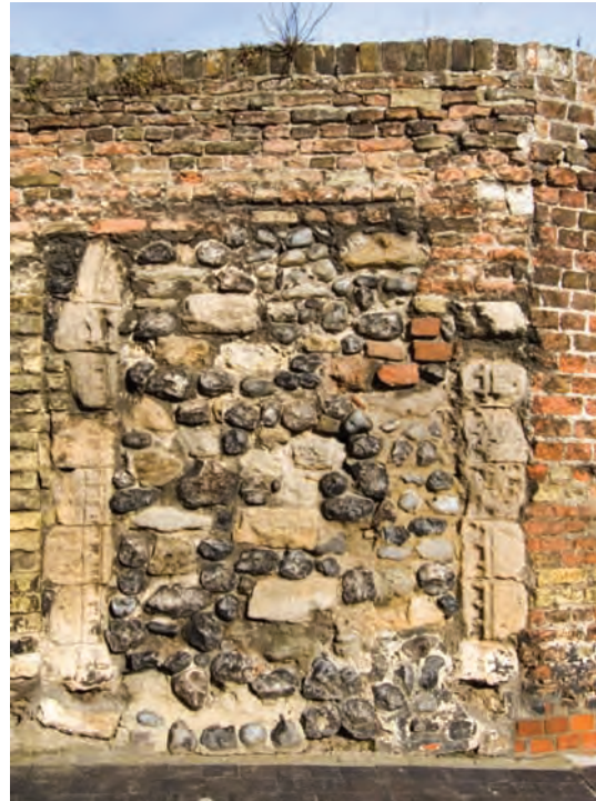
Fig. 7.16: Reset thirteenth-century doorway in Paradise Row (House 67) (P. W. © English Heritage DP043953)
