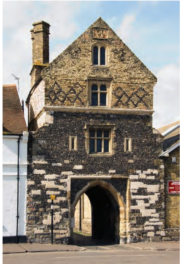
Fig. 11.18: The north face of Fisher Gate (P. W. © English Heritage DP026001)
