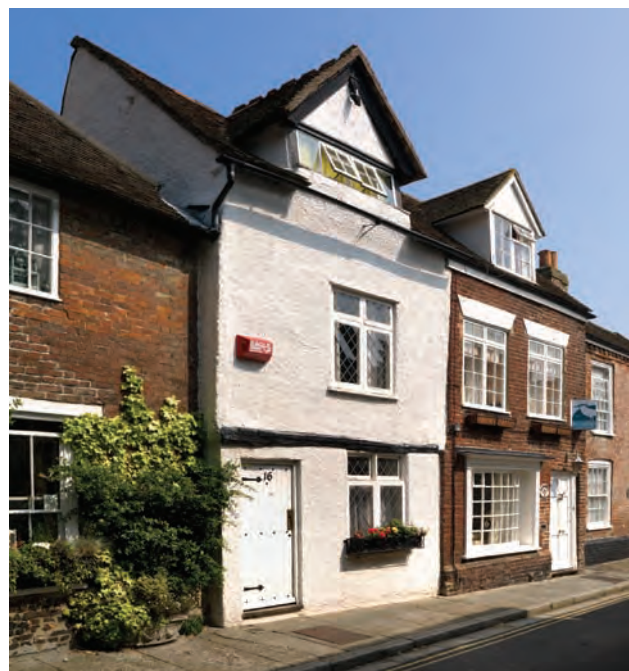
Fig. 16.29: 16 (and 14) St Peter's Street (House 69) (P. W. © English Heritage DP068617)
