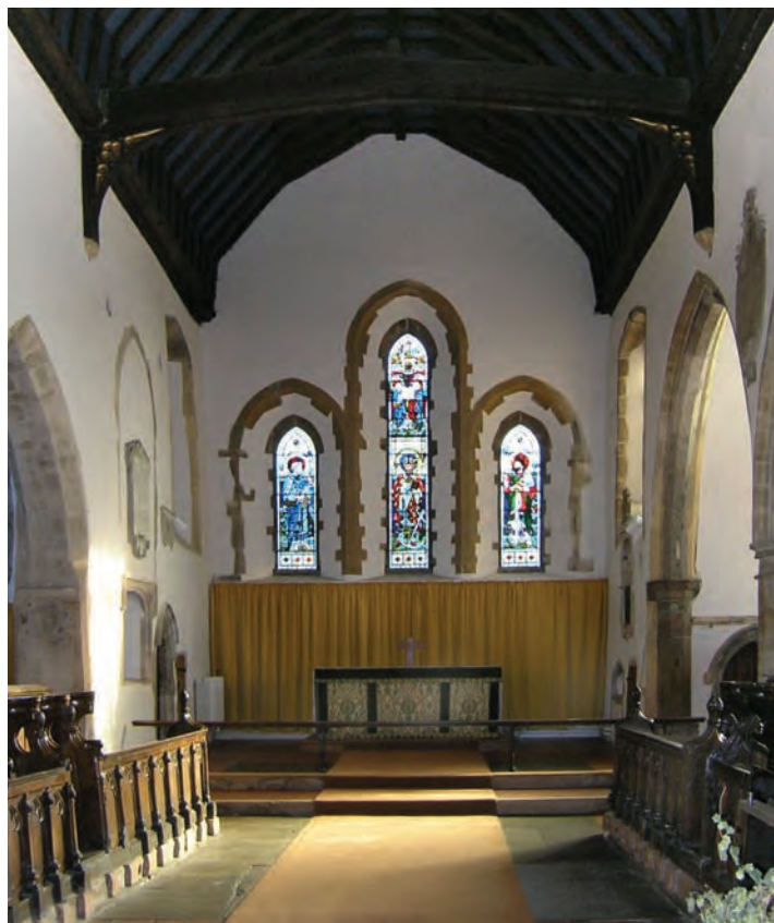
Fig. 6.2: St Clement's church, chancel, looking east to restored lancet windows and blocked lancet on north wall (S. P.)
