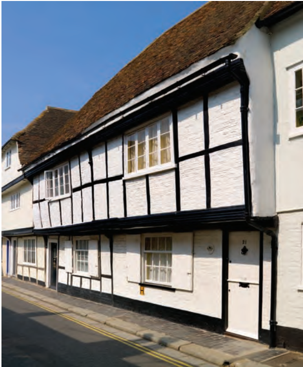
Fig. 16.24: 19, 21 Church Street St Mary (House 13), two single-bay houses, now of two storeys, but brackets at eaves level show where attic gables have been removed (P. W. © English Heritage DP068593)
