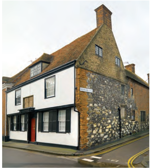
Fig. 16.14: Richborough House, 7 Bowling Street (House 2), from the east (P. W. © English Heritage DP032215)
