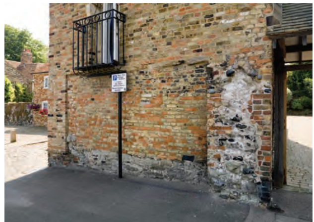
Fig. 11.25: Wall scars on the north face of the Round House (P. W. © DP068609)
