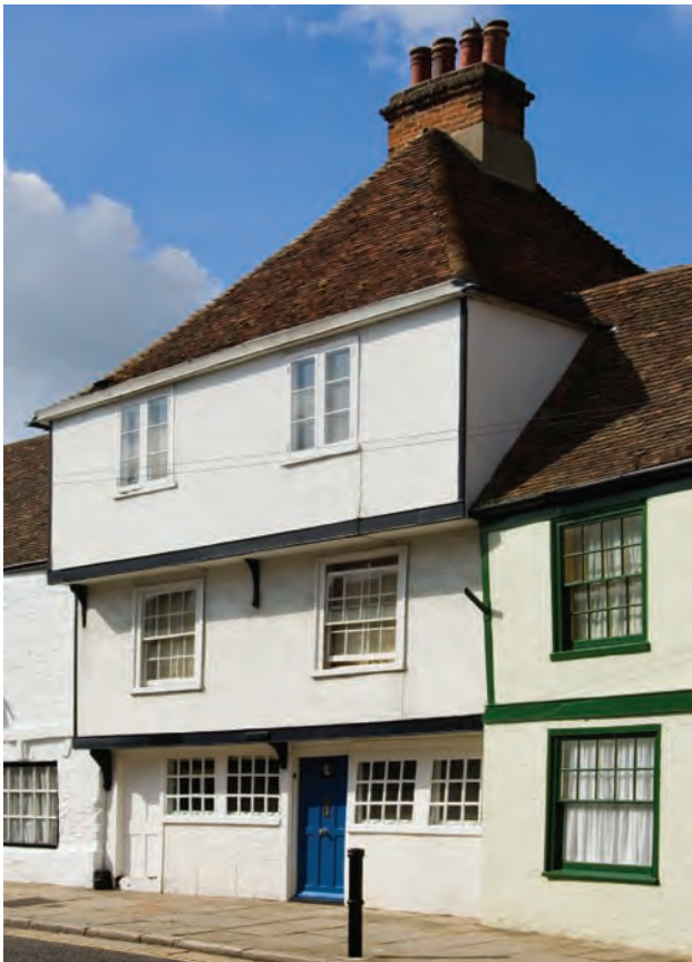
Fig. 16.22: 16, 18 New Street (House 63), view from north (P. W. © English Heritage DP044003)
