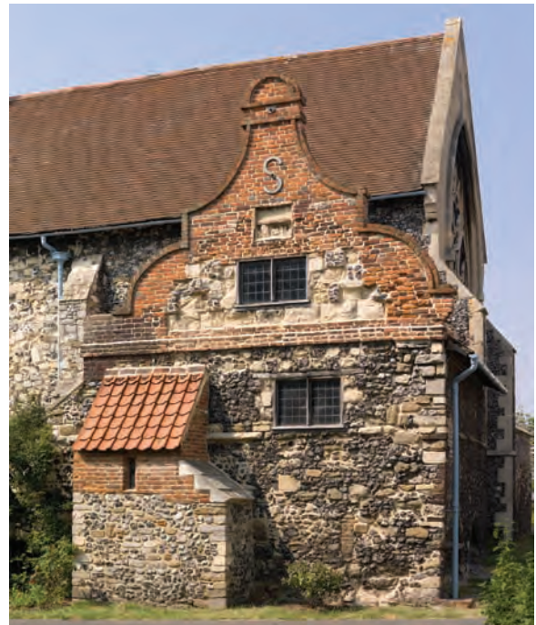
Fig. 6.14: St Peter's church, the extension at the east end of the south aisle: undercroft below and rebuilt first floor (P. W. © English Heritage DP068615)
