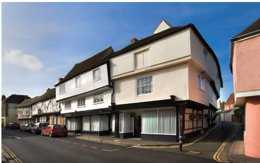
Fig. 12.4: Houses in Strand Street. From left to right: 11 (House 77); 13 and 15 (House 79); 19 and 21 (House 80); and 23 (House 81) Strand Street (P. W. © English Heritage DP043963)
