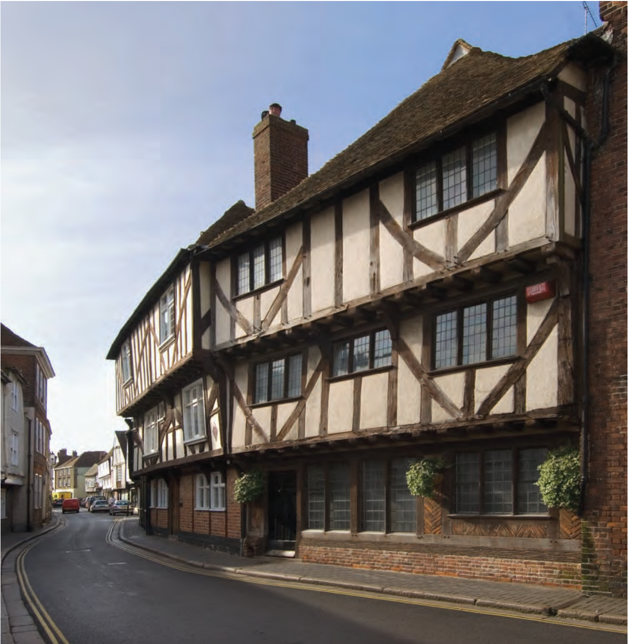
Fig. 7.20: 39 and 41 Strand Street from the north (Houses 85, 86) (P. W. © English Heritage DP043959)
