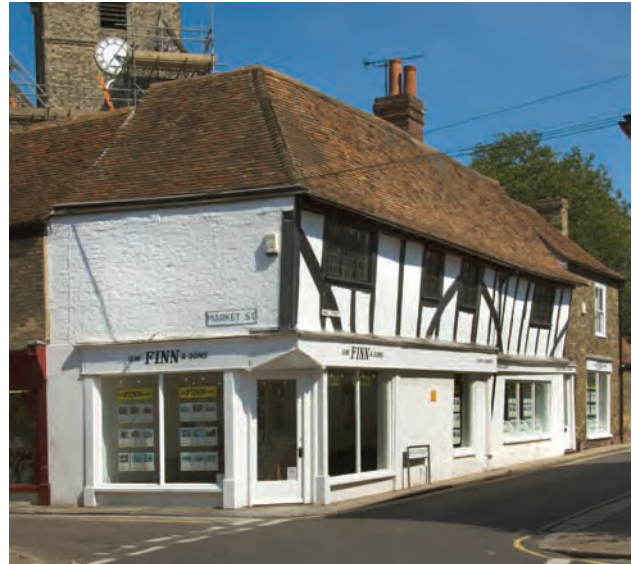
Fig. 12.45: 1, 3 King Street (Houses 41, 42), with St Peter's church behind (P. W. © English Heritage DP044036)
