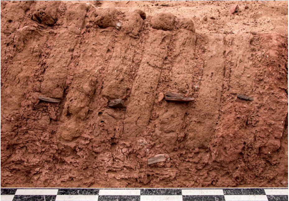
Fig. 5: Amheida: detail of the vault of room 14 in Serenos's house with chinking sherds.
