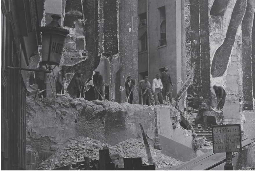
Fig. 3: Construction work to open up the Avenue de l'Opéra (1870–77) photograph by Charles Marville (excerpt).
