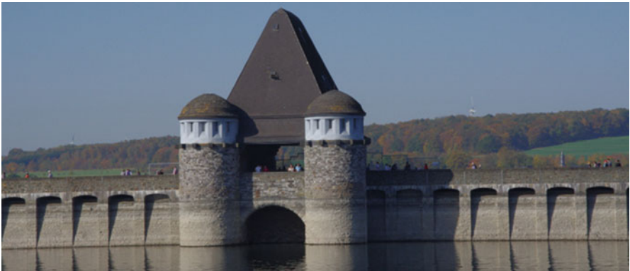
Fig. 1.4 Example of a dam to be monitored (Möhneseedamm), ©P. Marwedel
