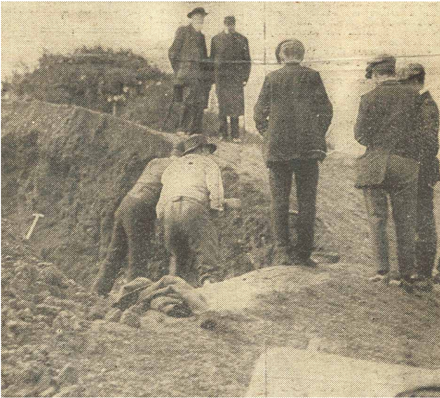
Figure 5.27. Excavation of Kings Hill, Bardney. Photo: Daily Graphic , 31st August 1912.
