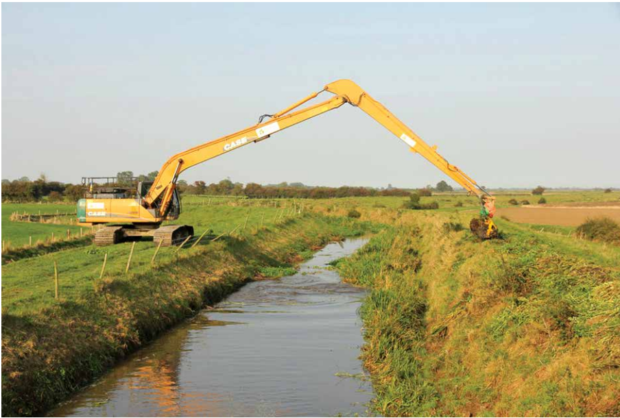
Figure 3.9. Dredging of the Great Eau at Withern. Image copyright Richard Croft. This work is licensed under Creative Commons Attribution-Share Alike 2.0 Generic Licence.
