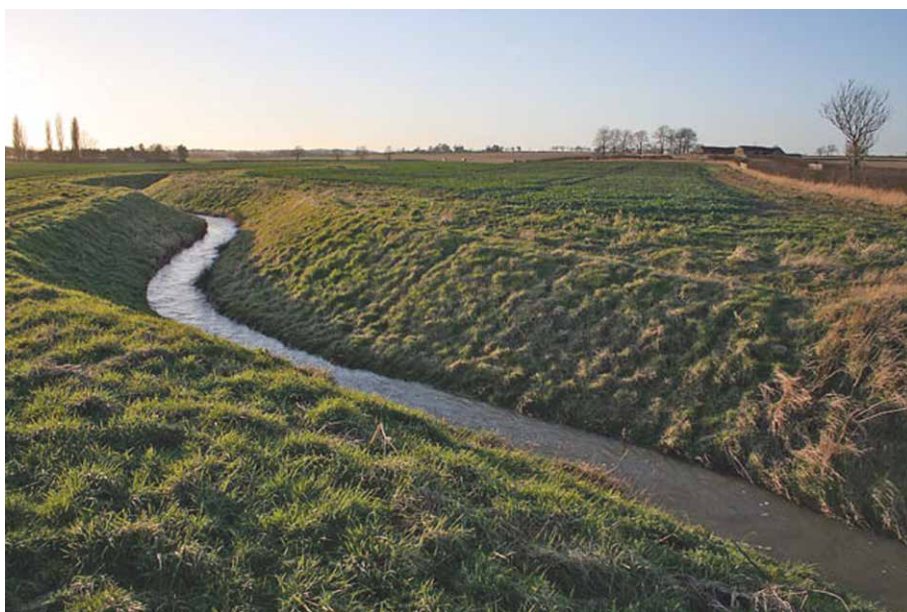
Figure 3.11. South Beck at Osbournby. The beck has been mechanically deepened and now cuts into underlying sands and gravels. Image copyright Kate Jewell. This work is licenced under the Creative Commons Attribution-Share Alike 2.0 Generic Licence.
