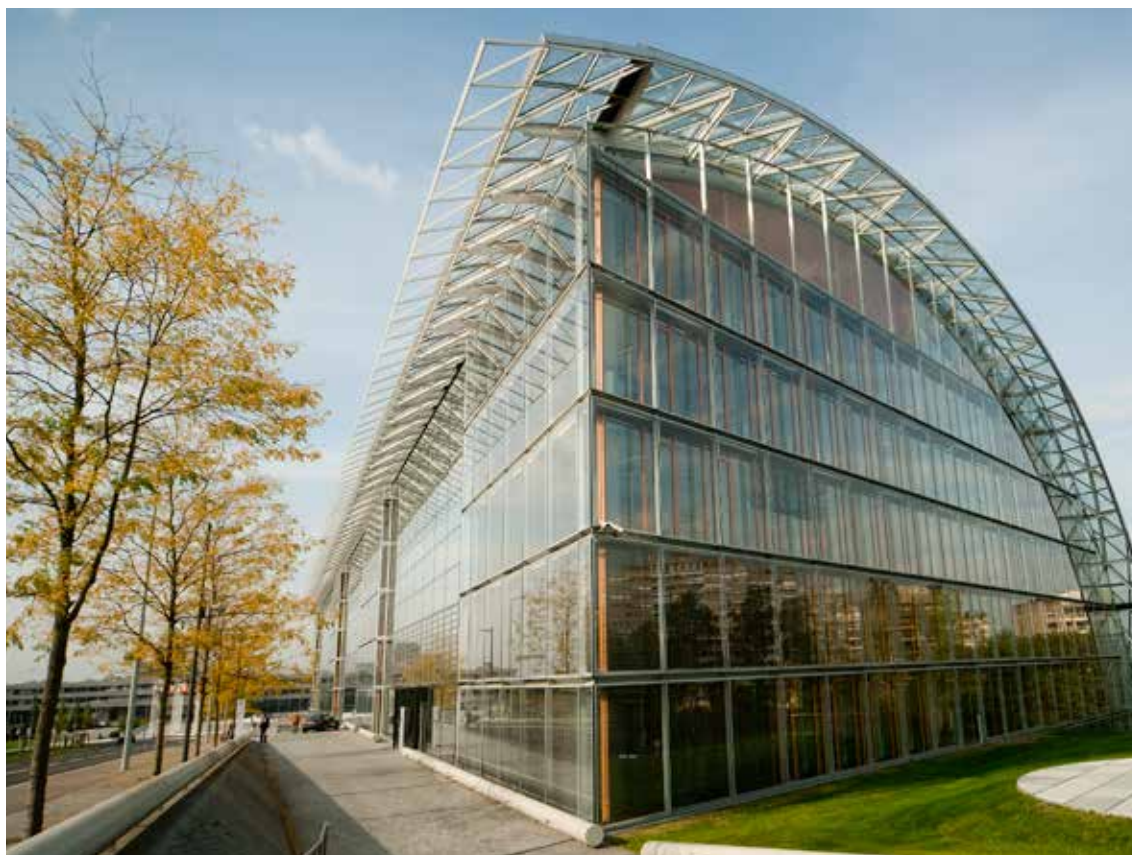
EIB EKI building
