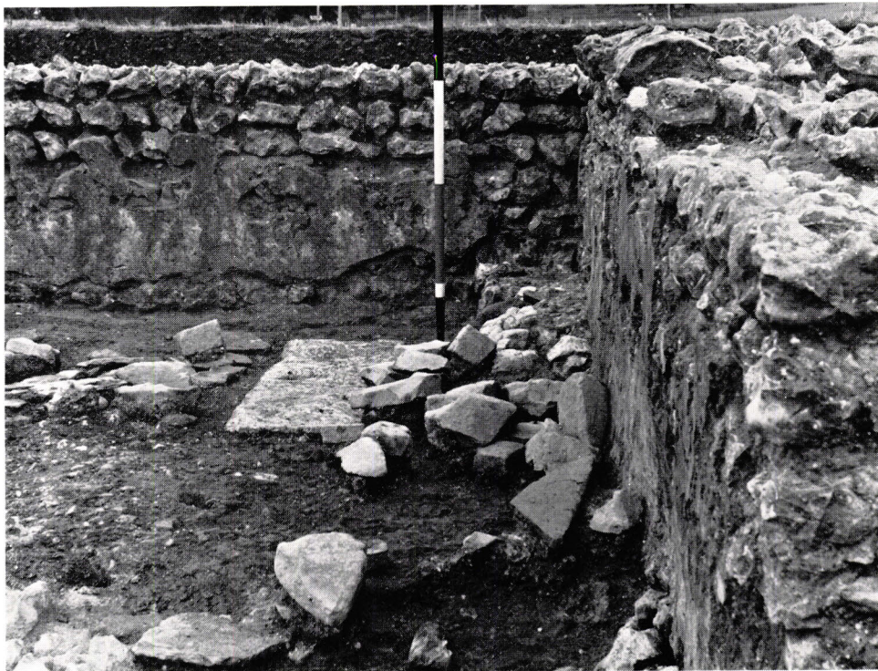
b. Oven in south-west corner of Room 20. Collapsed voussoirs in foreground. View south
