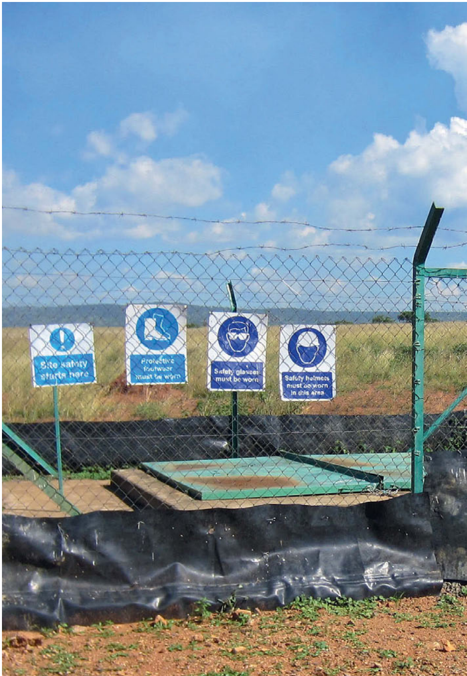
Figure 19: Closed well with safety warnings, Hoima district (2012).
